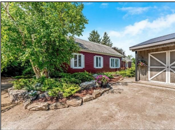
Figure 38: Side (northeast) elevation of the subject dwelling (HouseSigma 2021)
