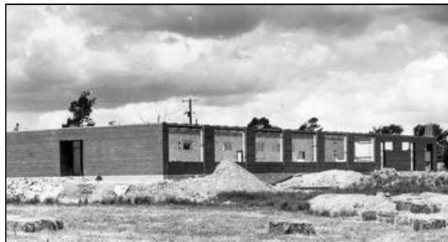
Figure 22: Construction of Pineview School, c. 1963 (EHS06426)
