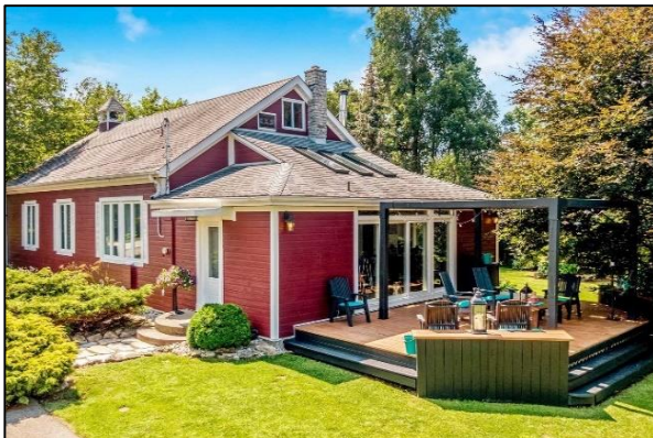
Figure 42: Partial rear (northwest) elevation of the subject dwelling (HouseSigma 2021)
