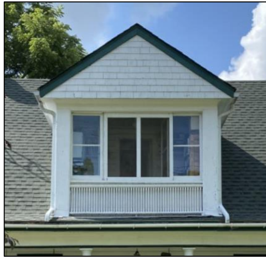
Figure 21: Central dormer along the front (southeast) elevation (Town of Halton Hills 2023)
