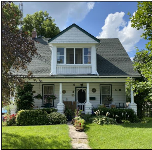
Figure 20: Front (southeast) elevation of the existing dwelling (Town of Halton Hills 2023)
