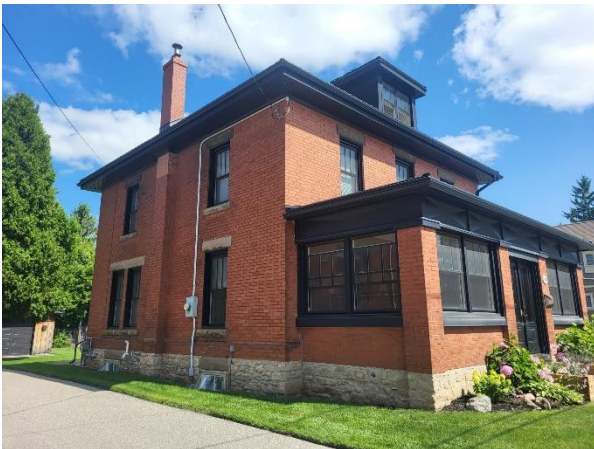
Figure 20: Southeast corner of the existing building at 93 Bower Street, showing the side (southwest) and front (southeast) elevations (Town of Halton Hills 2024)
