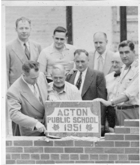
Figure 13: Cornerstone laid for the addition to Acton Public School, c.1951. Wolfe is pictured back left (Acton Free Press / Dills Collection courtesy Vintage Acton)
