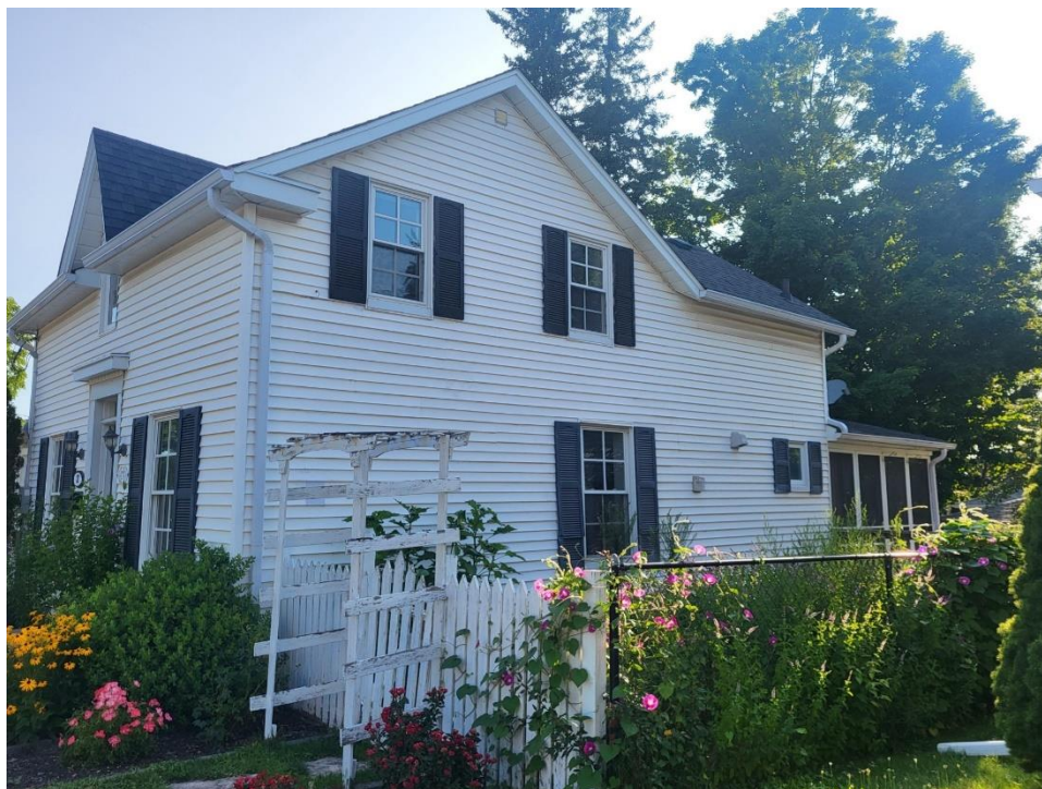
Figure 20: Side (south) elevation of the existing building at 12 Chapel Street (Town of Halton Hills 2024)
