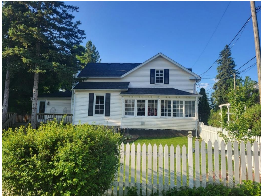
Figure 19: Side (north) elevation of the existing building at 12 Chapel Street (Town of Halton Hills 2024)
