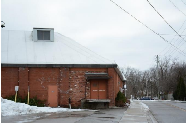
Figure 37: Detail of the south end of the west elevation (Town of Halton Hills 2023)
