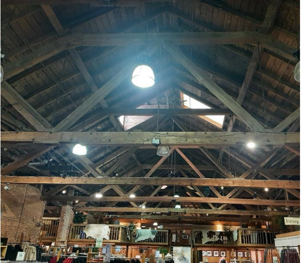
Figure 38: Interior roof structure within the Hide House (Heritage Halton Hills 2024)
