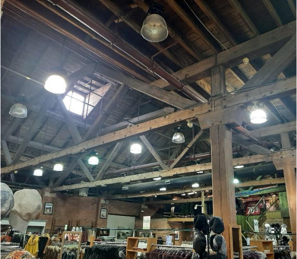
Figure 39: Interior roof structure within the Hide House (Heritage Halton Hills 2024)
