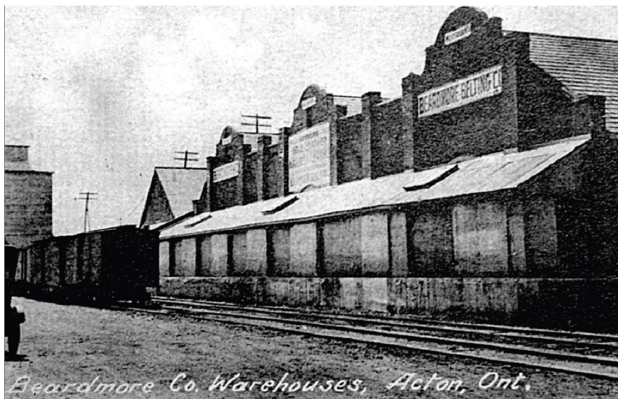
Figure 9: North facade of the Hide House, n.d. (The New Tanner 2006)
