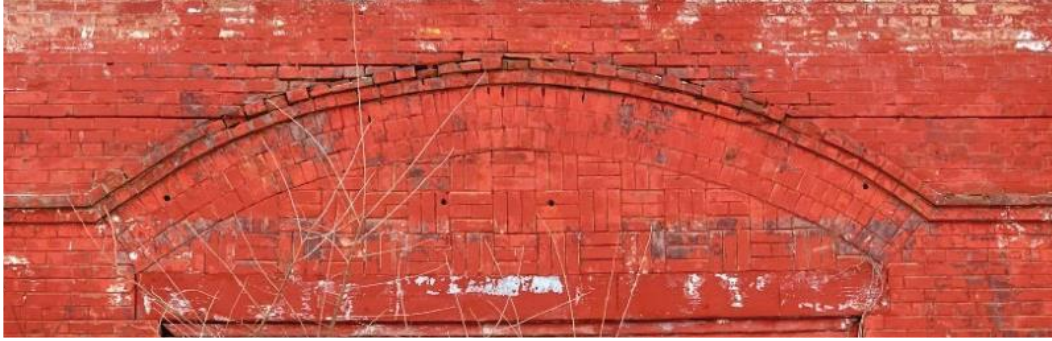
Figure 30: Detail of the basketweave brickwork on the north elevation (Metrolinx 2022)
