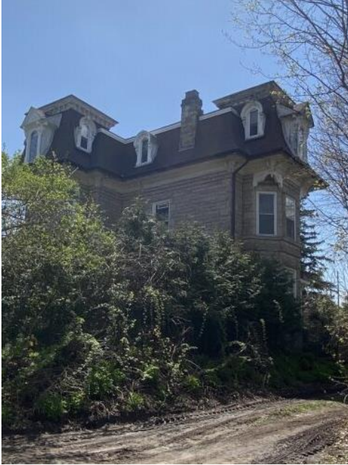
Figure 22: Partial side (southeast) elevation of Grey Vernon (Town of Halton Hills 2024)
