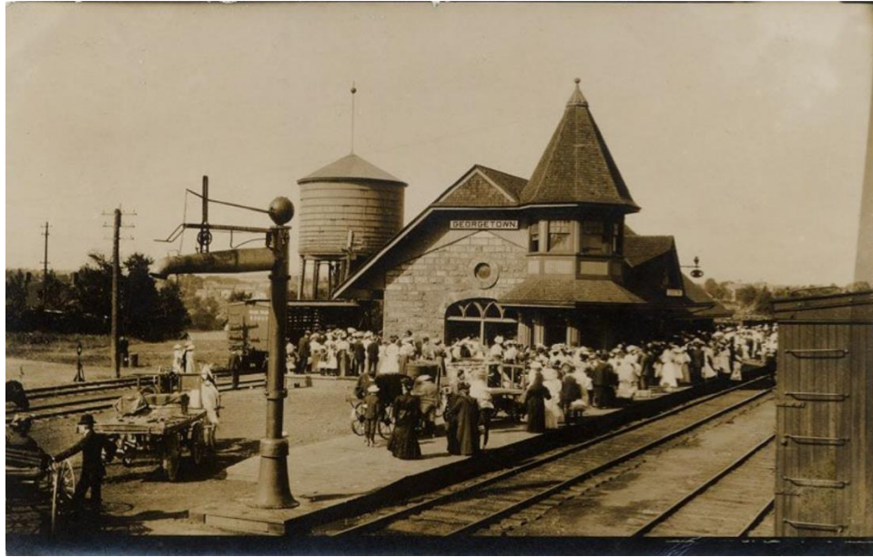
Figure 7: A crowd waits for the train outside the Grand Trunk Railway Station in Georgetown, c.1908 (EHS p315f)
