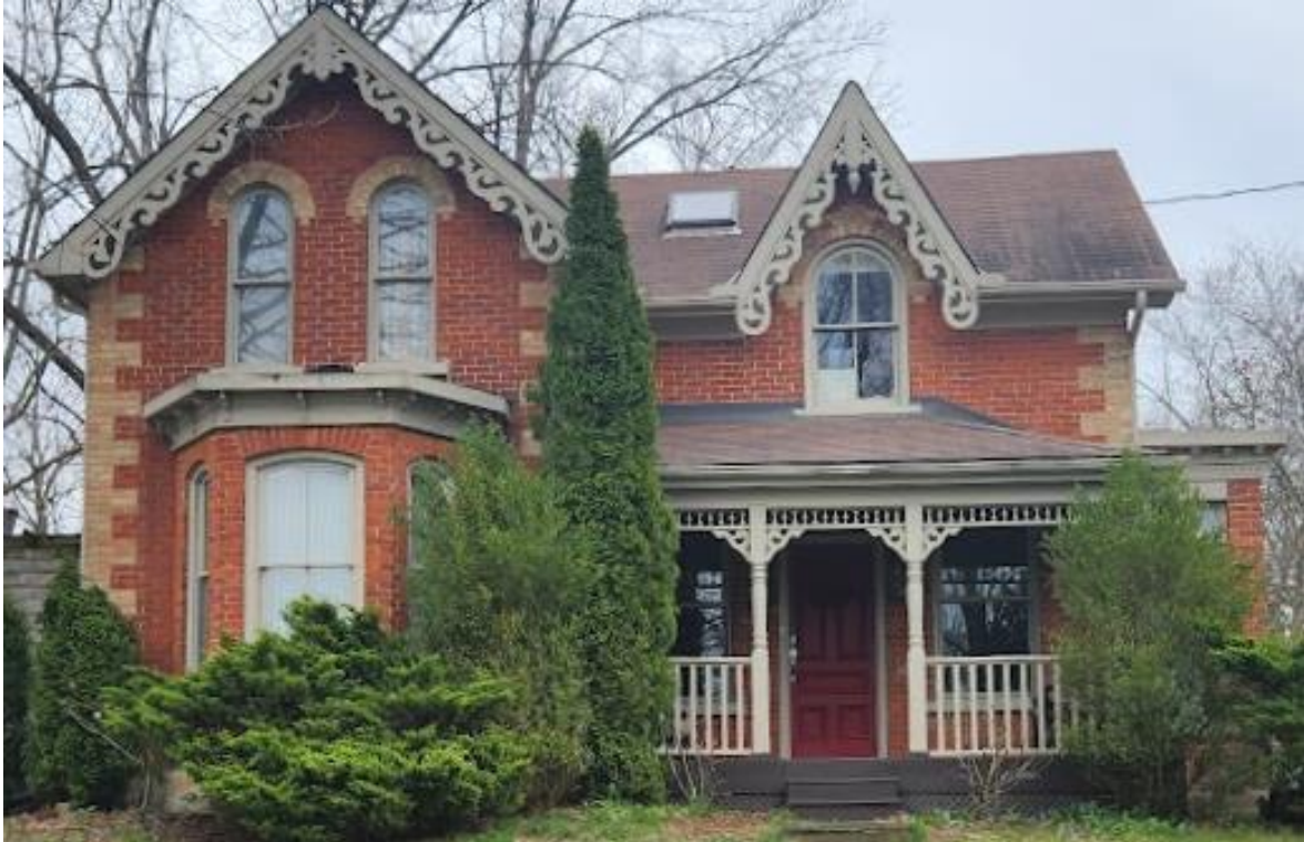
Figure 24: Front (northwest) elevation of the existing building at 14-16 Queen Street (Town of Halton Hills 2024)
