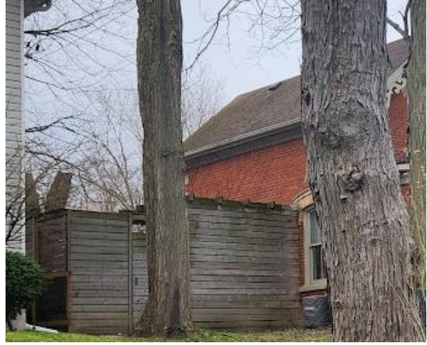
Figure 26: Partial northeast elevation of the existing building (Town of Halton Hills 2024)
