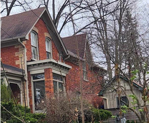
Figure 25: Partial southeast elevation of the existing building (Town of Halton Hills 2024)
