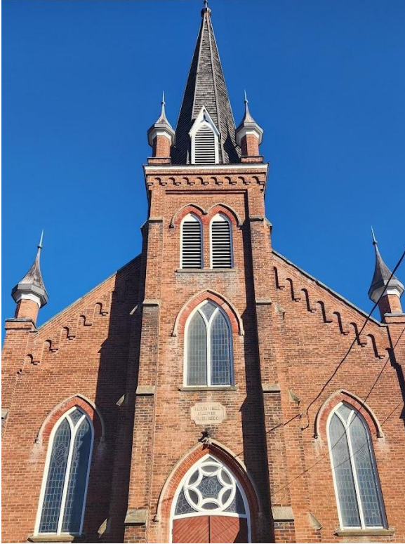
Figure 34: Detail of front (south) elevation of Norval Presbyterian Church (Town of Halton Hills 2024)
