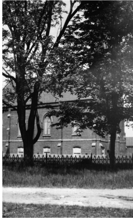
Figure 12: Norval Presbyterian Church as seen from Draper Street, c.1935 (EHS 20708)
