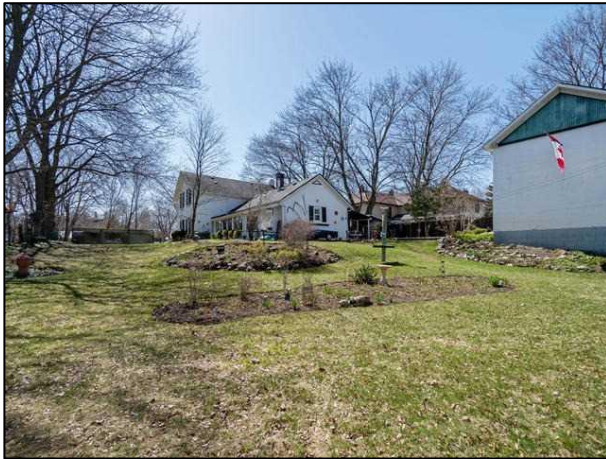
Figure 24: Looking towards the southeast and northeast elevations of the dwelling (Housesigma 2018)
