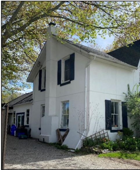
Figure 20: West corner of the existing dwelling (Town of Halton Hills 2024)
