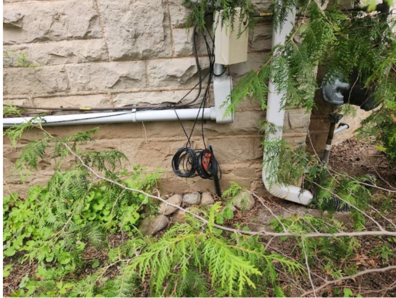
Figure 35: Detail of the side (northeast) elevation of UENI at 22 Queen Street, showing the stone foundation (Town of Halton Hills 2024)
