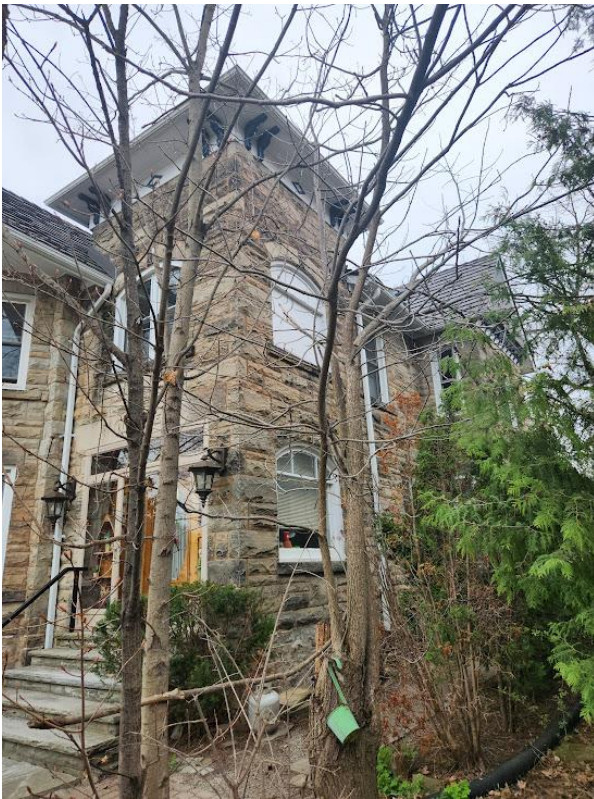
Figure 37: West corner of ILLAHEE at 24 Queen Street, partially obscured (Town of Halton Hills 2024)
