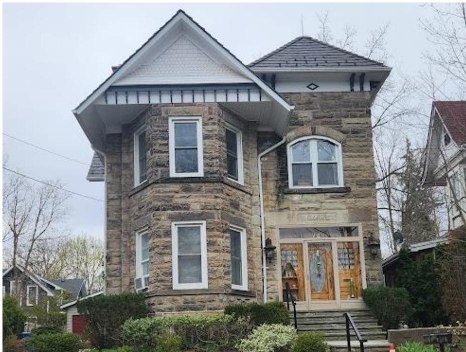
Figure 36: Front (northwest) elevation of ILLAHEE at 24 Queen Street (Town of Halton Hills 2024)
