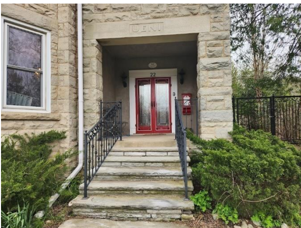
Figure 26: Detail of the front (northwest) elevation of UENI at 22 Queen Street (Town of Halton Hills 2024)
