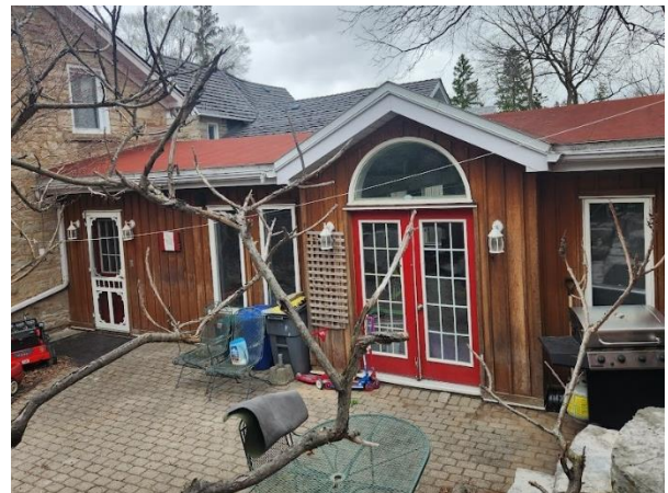
Figure 30: Looking at the south corner of UENI at 22 Queen Street, showing the one-storey rear addition (Town of Halton Hills 2024)
