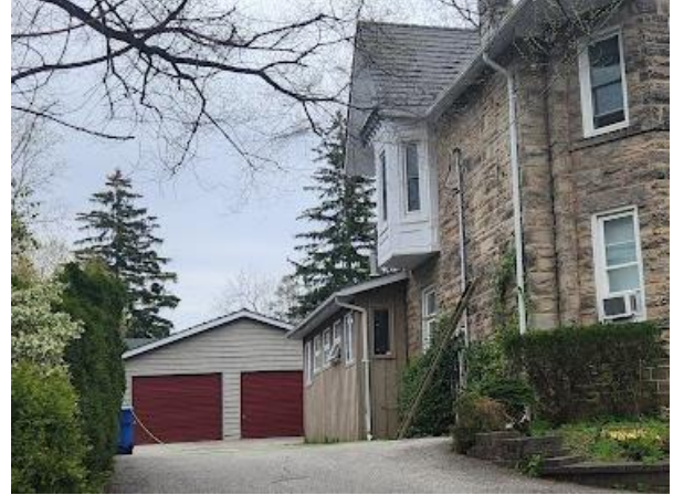
Figure 40: Partial side (northeast) elevation of ILLAHEE at 24 Queen Street (Town of Halton Hills 2024)
