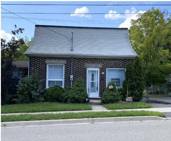
Figure 16: Former coal depot, now residence, at 45 Queen Street (Town of Halton Hills 2023)
