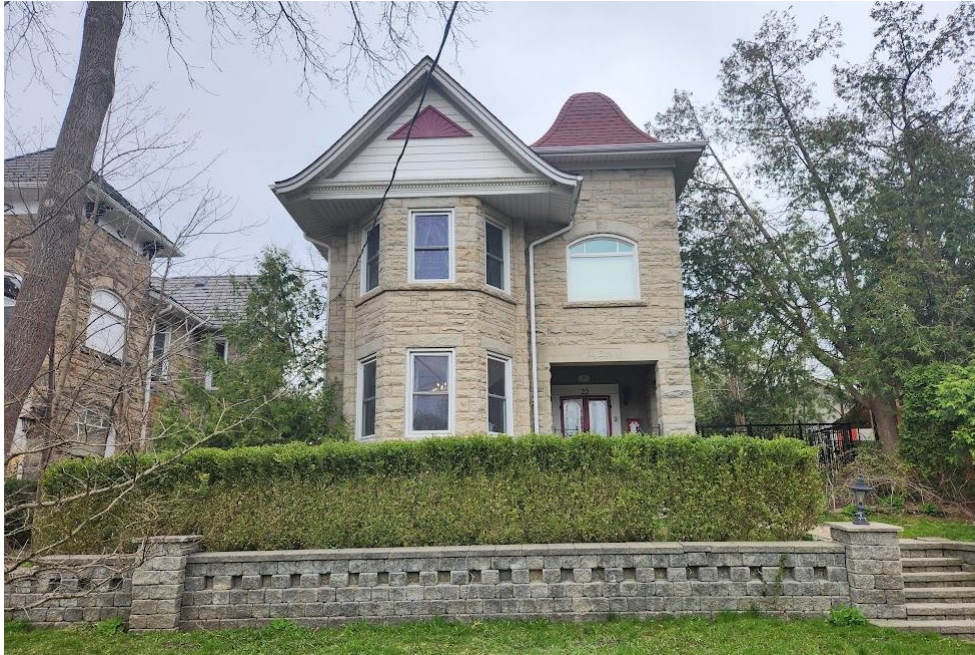
Figure 25: Looking towards UENI at 22 Queen Street from the sidewalk along Queen Street (Town of Halton Hills 2024)
