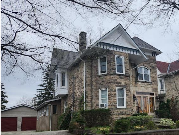
Figure 39: Looking towards the north corner of ILLAHEE at 24 Queen Street (Town of Halton Hills 2024)
