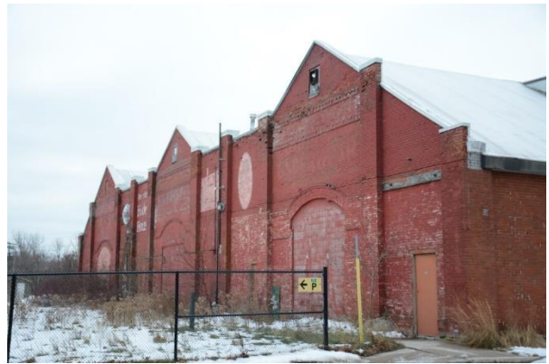
Figure 27: Looking along the north elevation of the Hide House from within the existing parking lot (Town of Halton Hills 2023)
