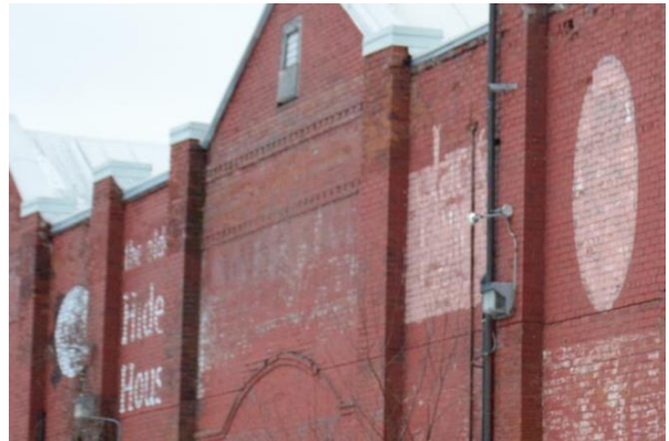
Figure 29: Detail of the north elevation showing the brick pilasters, brick detailing and remnant advertisements (Town of Halton Hills 2023)
