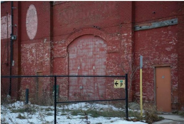
Figure 28: Detail of the north elevation showing the brick pilasters, brick detailing and remnant advertisements (Town of Halton Hills 2023)
