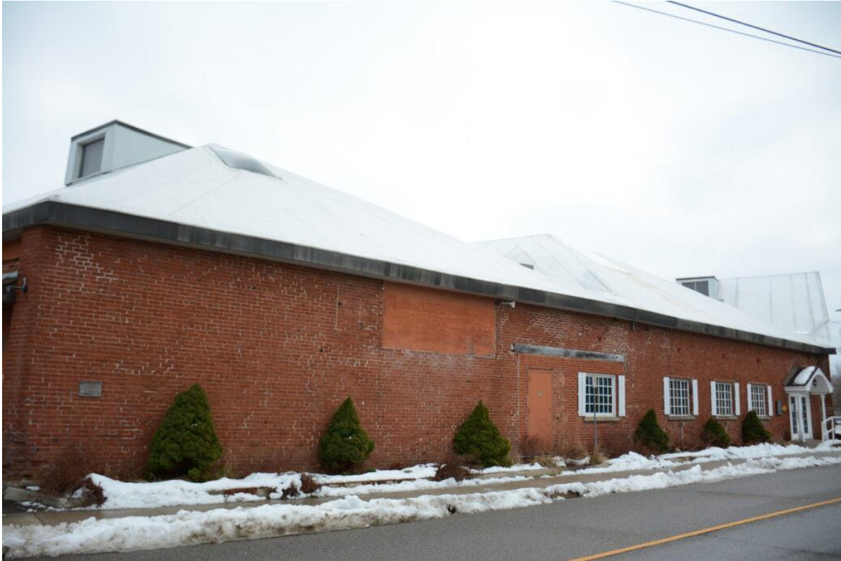
Figure 33: West end of the south elevation along Eastern Avenue (Town of Halton Hills 2023)
