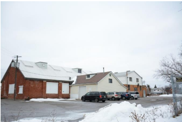
Figure 31: East elevation from Eastern Avenue (Town of Halton Hills 2023)
