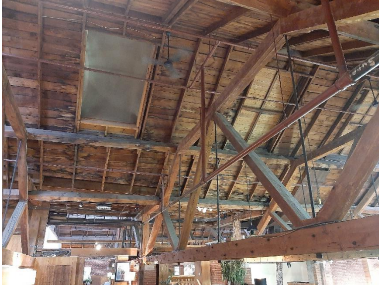
Figure 40: Interior roof structure within the Hide House (Heritage Halton Hills 2024)
