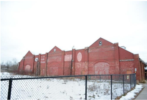
Figure 26: North elevation of the Hide House (Town of Halton Hills 2023)
