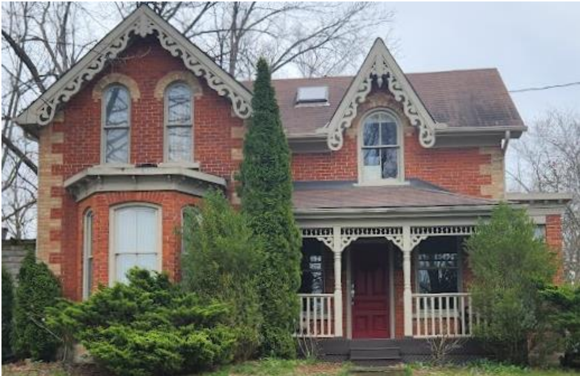
Figure 24: Front (northwest) elevation of the existing building at 14-16 Queen Street (Town of Halton Hills 2024)
