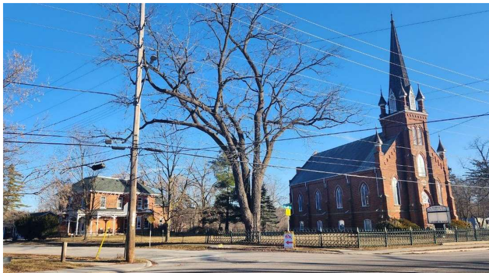
Figure 31: Looking northeast towards the Norval Presbyterian Church (right) and Norval Presbyterian Manse and Cottage (left) (Town of Halton Hills 2024)
