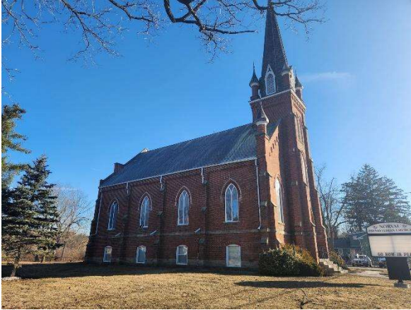
Figure 36: Side (west) elevation of Norval Presbyterian Church (Town of Halton Hills 2024)
