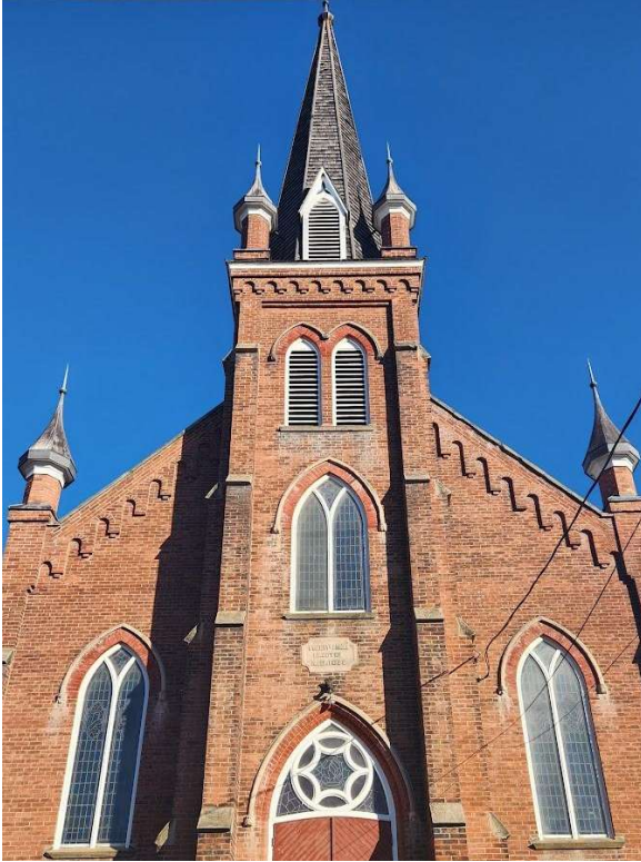
Figure 34: Detail of front (south) elevation of Norval Presbyterian Church (Town of Halton Hills 2024)
