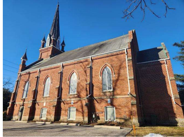
Figure 37: Side (east) elevation of Norval Presbyterian Church (Town of Halton Hills 2024)
