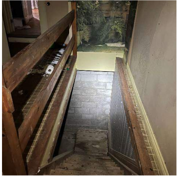
Staircase to Basement
