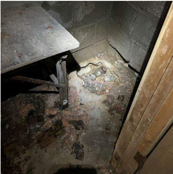
Basement Storage Room with Buckling Concrete Block Foundation
