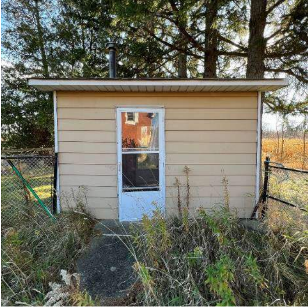
West Façade of Pool Shed
