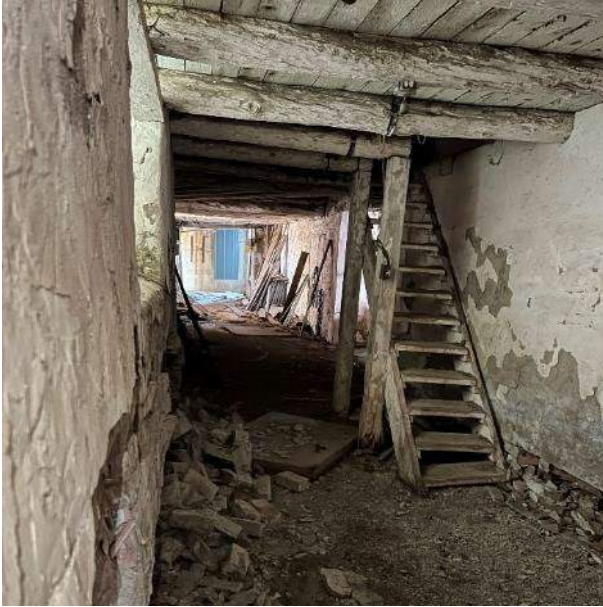
Central Hallway and Staircase to Upper Level
