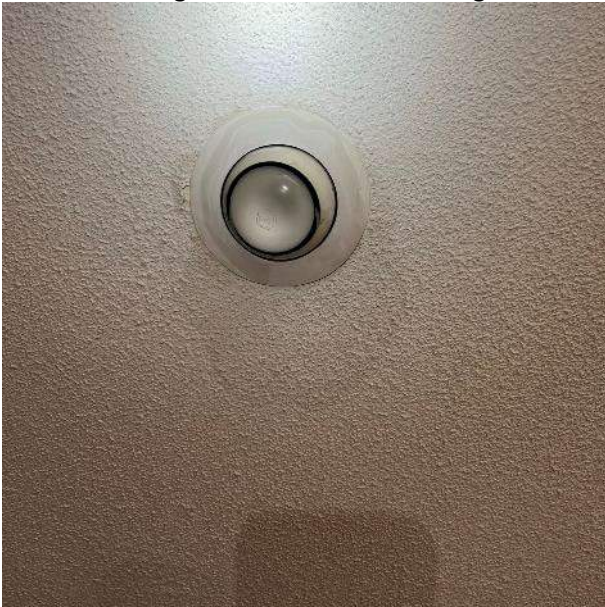
Pot Light with Water Damage
