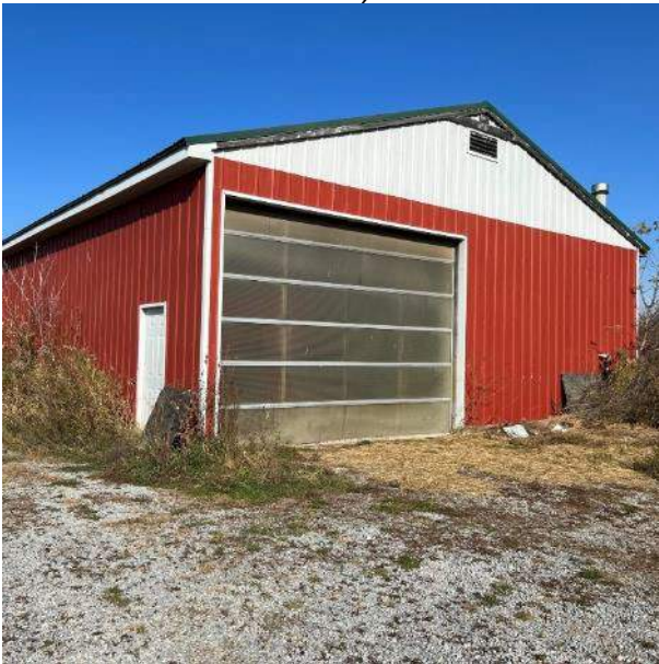
Southeast Facade of Outbuilding (Drive Shed)
