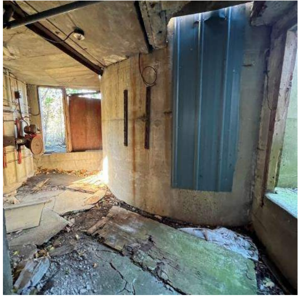
Connection with Concrete Silo
