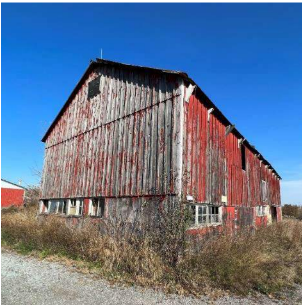
South Corner Façade of Smaller Barn
