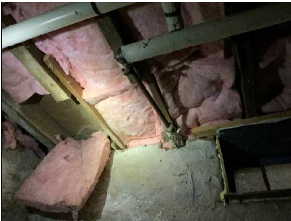
Photograph 4: Cut joists.
