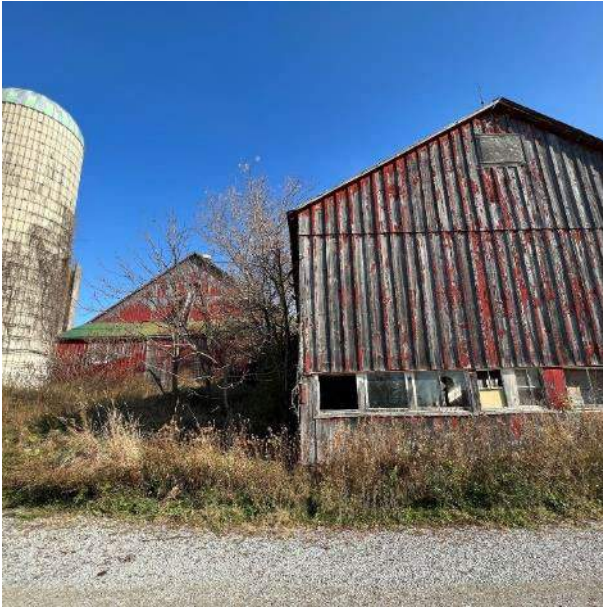
Southwest Facades of Both Barns
