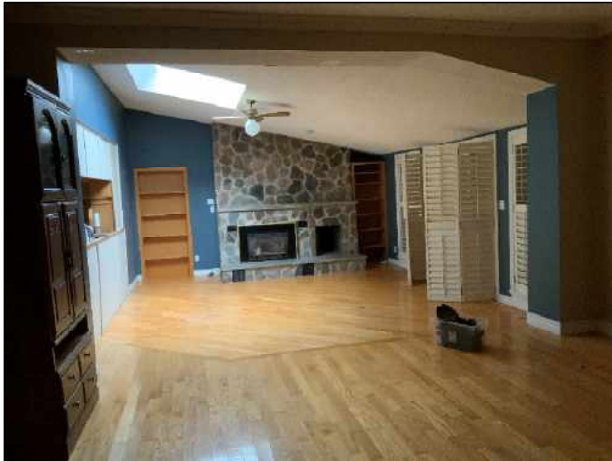
Photograph 3: Overview of living room addition.
