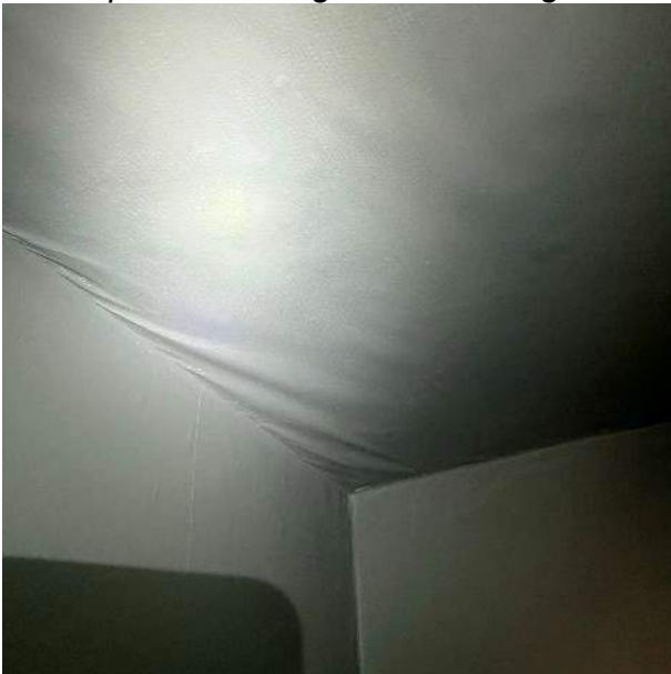
Upstairs Ceiling Water Damage
