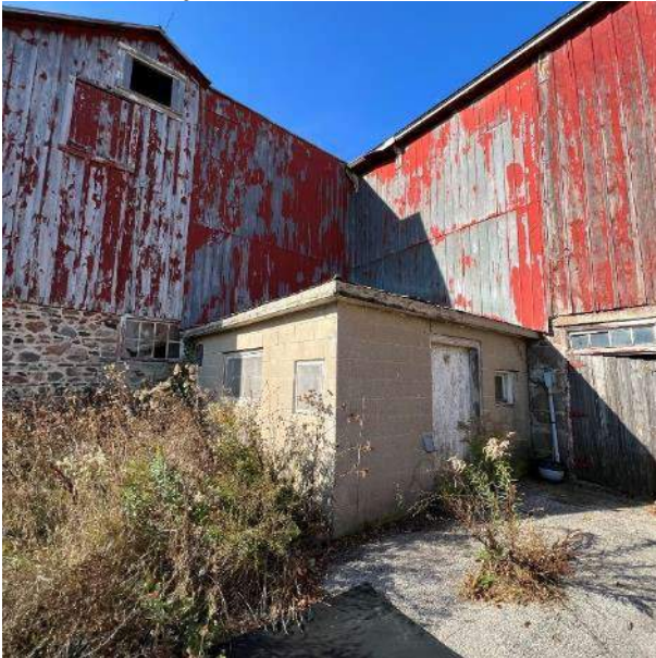
1-Storey Concrete Block Addition
