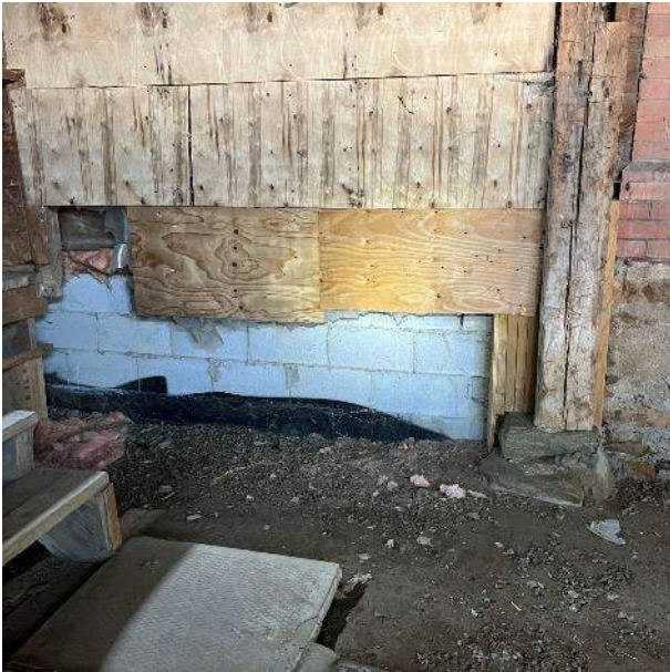
Garage Addition Concrete Block Foundation Walls
