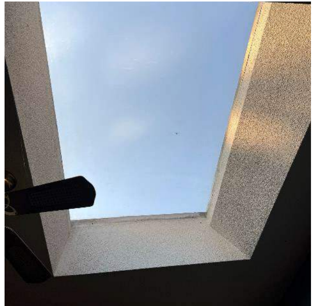
Skylight in Living Room Addition
