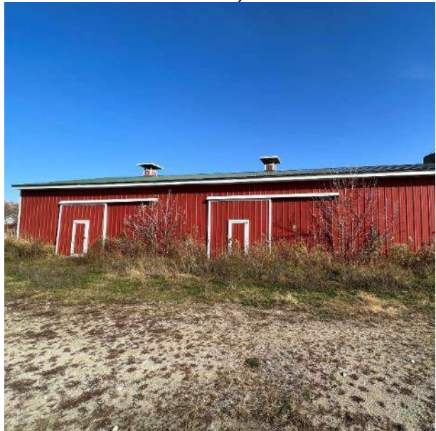
Southwest Façade of Outbuilding (Drive Shed)
