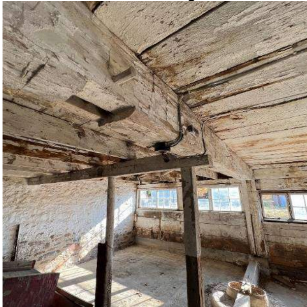
Mortise and Tenon Joints Secured by Wooden Pegs
