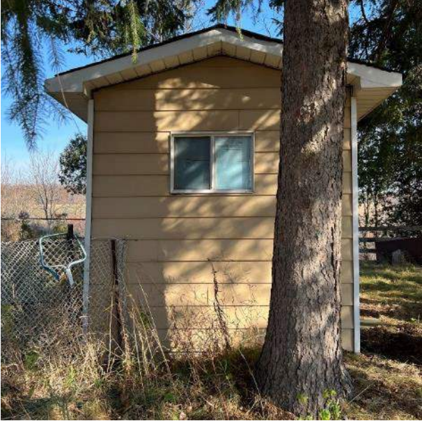
South Façade of Pool Shed
