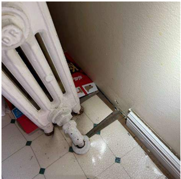
Radiator and Peeling Linoleum Flooring
