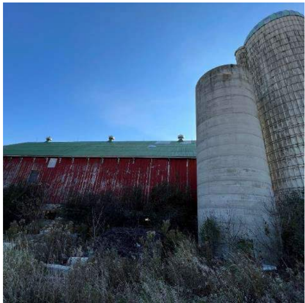
Northwest Façade of Larger Barn with Silos
