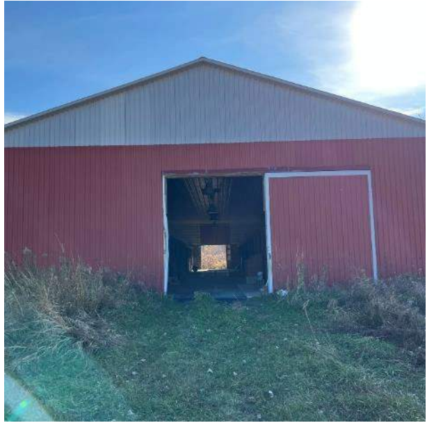
Northwest Entrance to Stable Barn
