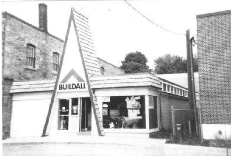
Figure 22: Mackenzie Lumber Buildall, c.1970 (EHS 08547)
