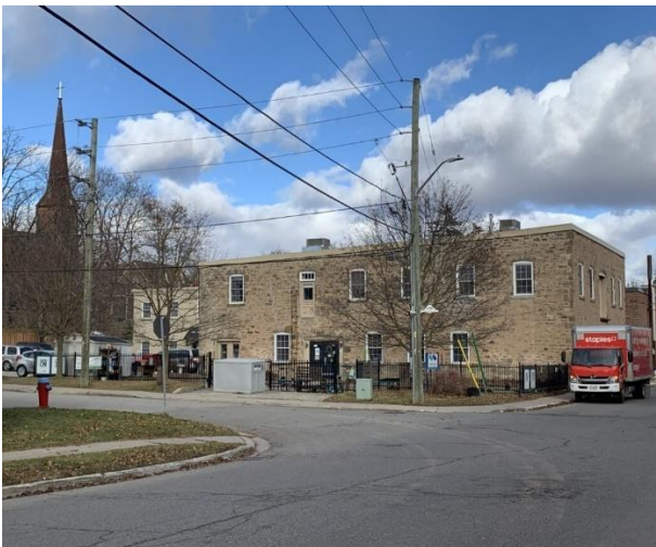
Figure 33: Looking towards the subject property from James Street (Town of Halton Hills 2023)
