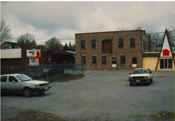
Figure 28: Mackenzie's Sawmill (Georgetown Lumber); front view, c.1988 (EHS 10750)
