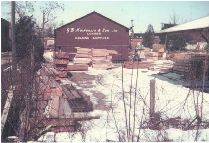
Figure 18: A winter view of the lumber yard for Mackenzie Lumber, c. 1955 (EHS 22696)
