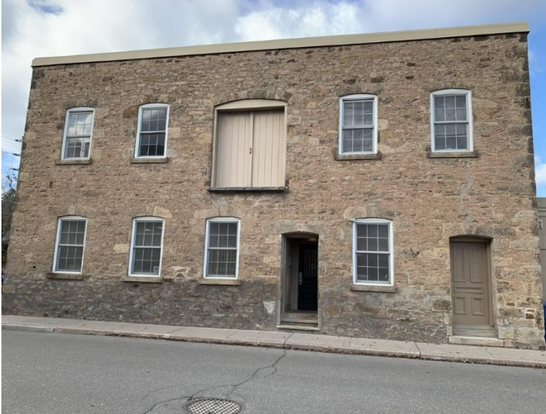
Figure 35: Primary (southeast) elevation of 8 James Street (Town of Halton Hills 2023)
