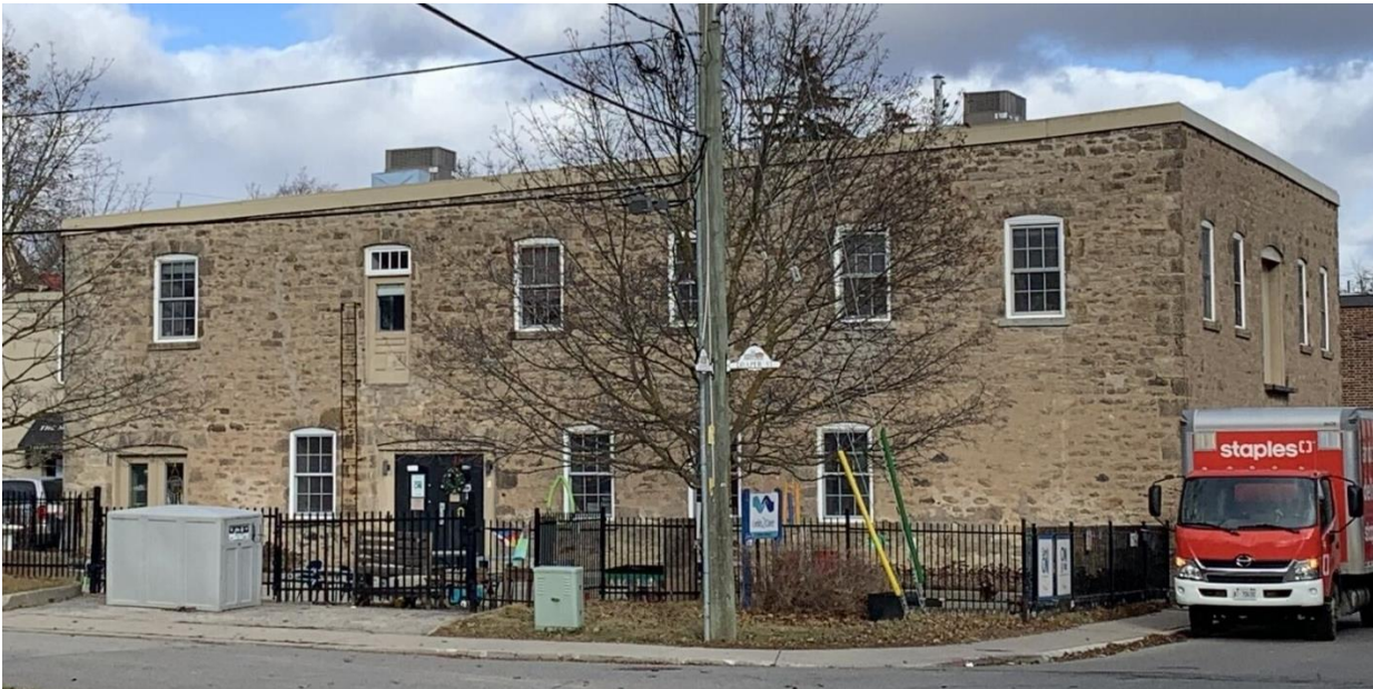
Figure 37: Southwest elevation of the existing building (Town of Halton Hills 2023)
