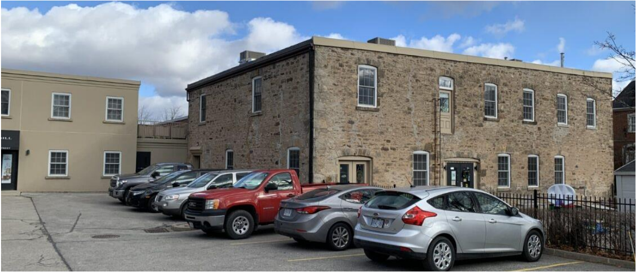
Figure 38: Northwest elevation of the existing building (Town of Halton Hills 2023)
