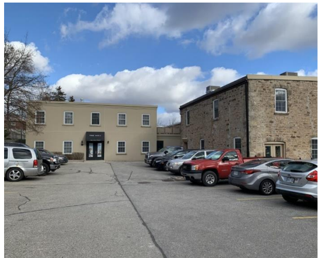
Figure 34: Looking from Draper Street towards the c.1897 stone building (Town of Halton Hills 2023)
