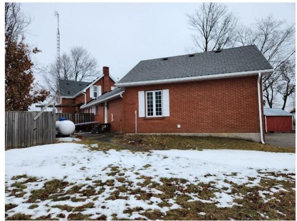
Figure 32: Looking towards the northeast elevation of the existing residence, showing the rear addition (Town of Halton Hills 2024)
