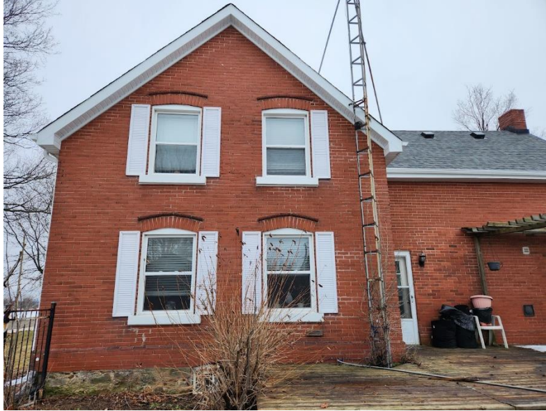
Figure 30: Partial northeast elevation of the existing residence (Town of Halton Hills 2024)
