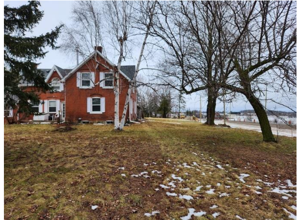
Figure 23: Looking northwest along Trafalgar at 9156 Trafalgar Road (Town of Halton Hills 2024)
