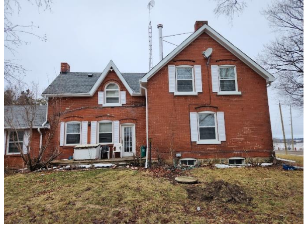
Figure 27: Partial southeast elevation of the existing residence (Town of Halton Hills 2024)
