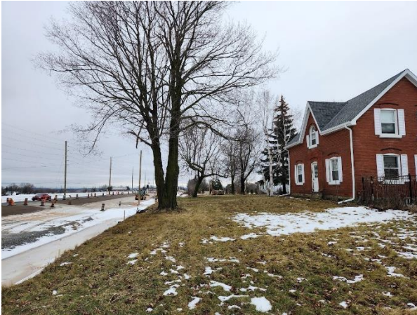
Figure 22: Looking southeast along Trafalgar at 9156 Trafalgar Road (Town of Halton Hills 2024)
