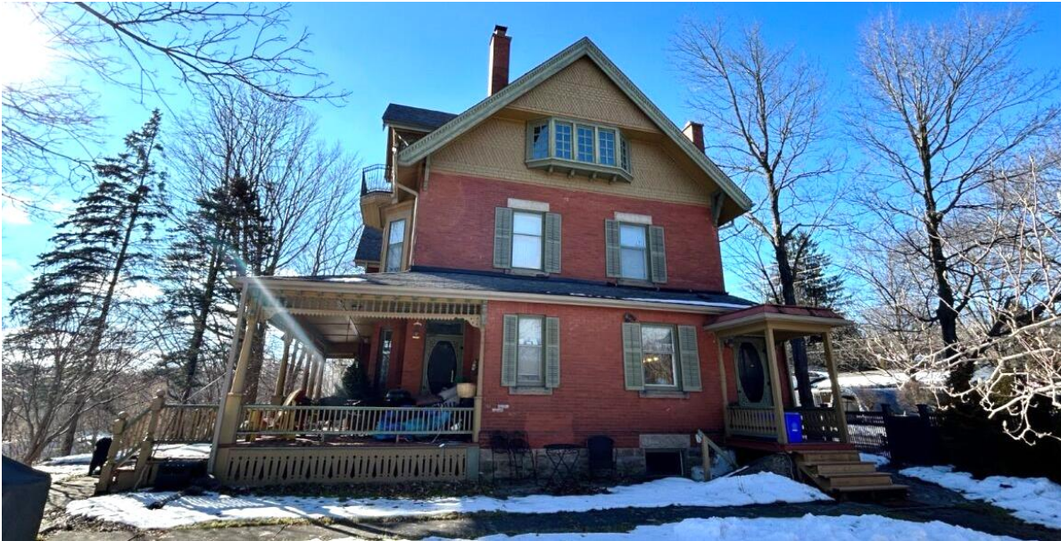
Figure 42: Northeast elevation of Barraclough House (Property Owner 2024)
