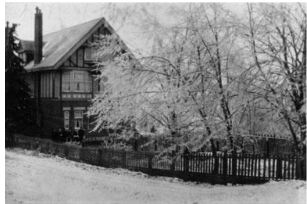
Figure 13: Barraclough House after an ice storm, c.1910 (EHS 00670)
