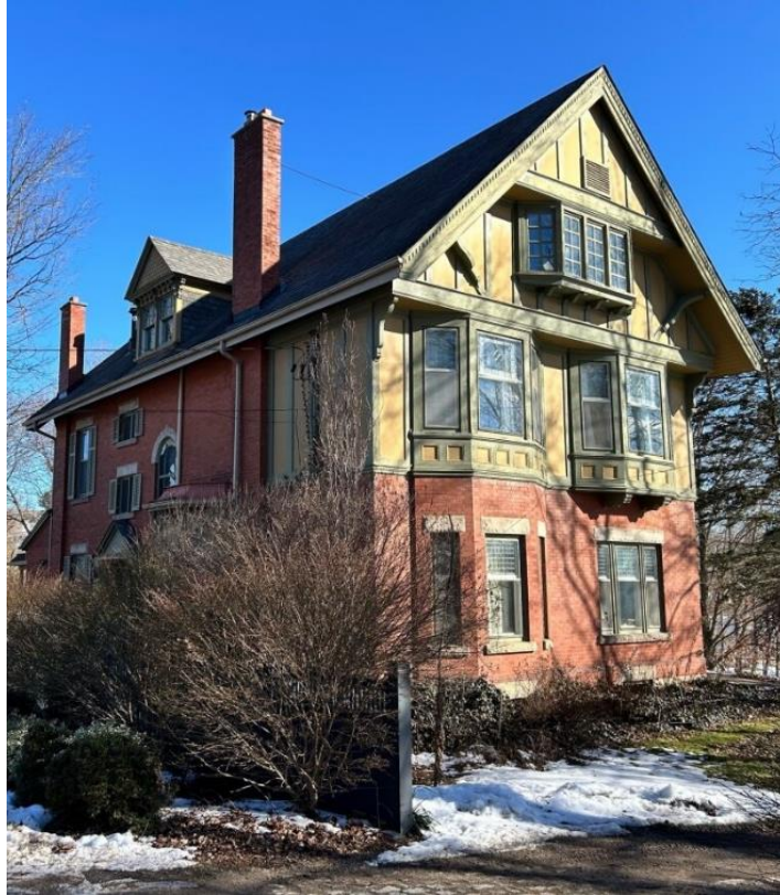
Figure 38: Southwest corner of Barraclough House (Property Owner 2024)
