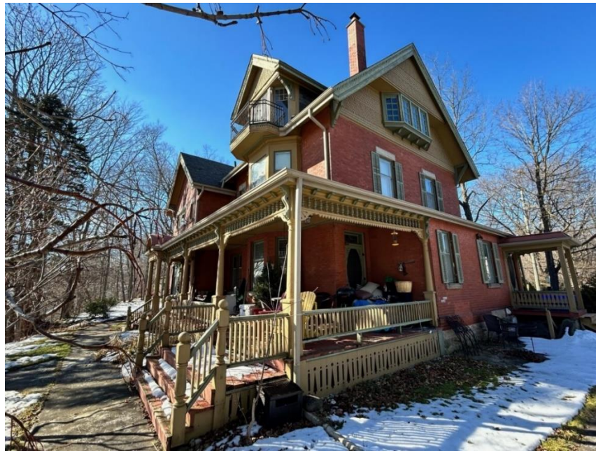
Figure 41: Southeast corner of Barraclough House (Property Owner 2024)
