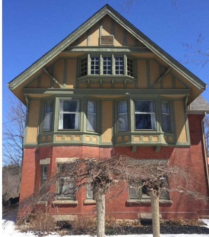
Figure 39: Southwest elevation of Barraclough House (Owner 2024)
