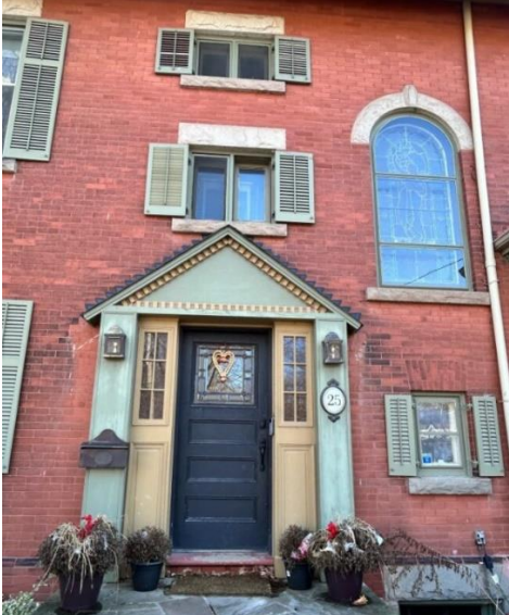
Figure 35: Detail of the front (north) elevation of Barraclough House (Property Owner 2024)
