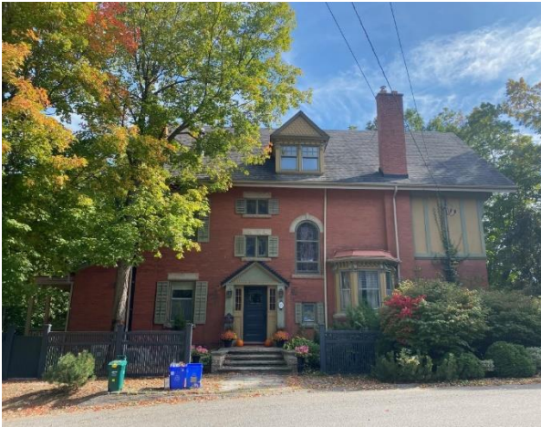
Figure 33: Front (north) elevation of Barraclough House at 25 Mountain Street, partially obscured by foliage (Town of Halton Hills 2023)
