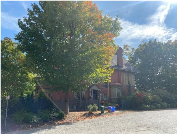
Figure 30: Looking south towards 25 Mountain Street from Tweedle Street, partially obscured by foliage (Town of Halton Hills 2023)
