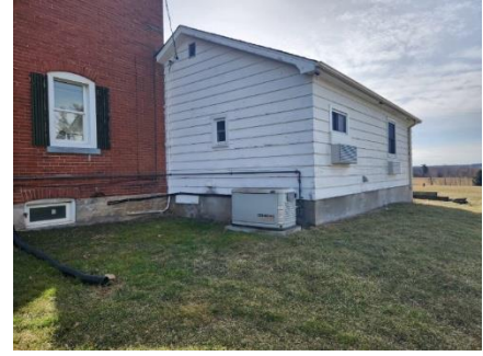
Figure 43: Looking towards the one-storey garage addition (Town of Halton Hills 2024)
