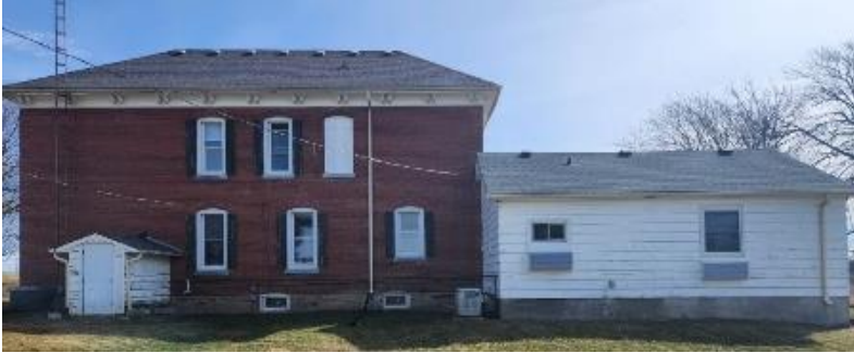
Figure 42: Northwest elevation with one-storey garage addition (Town of Halton Hills 2024)
