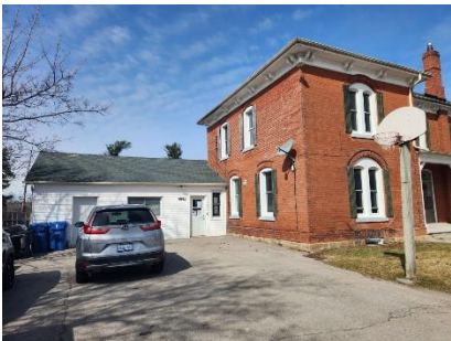
Figure 39: Looking towards the southwest corner with one-storey attached garage (Town of Halton Hills 2024)
