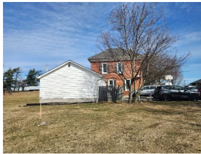
Figure 40: Southwest elevation with rear of the one-storey garage (Town of Halton Hills 2024)
