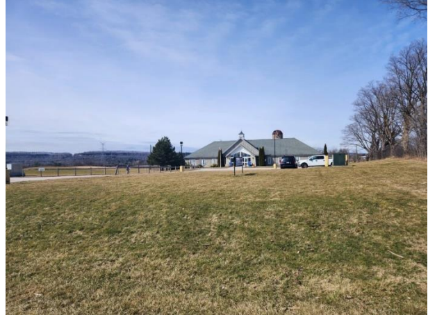
Figure 34: Looking northwest towards the Bob Rumball Centre within the southwest corner of the subject property (Town of Halton Hills 2024)
