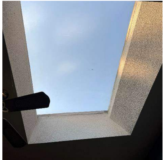
Skylight in Living Room Addition
