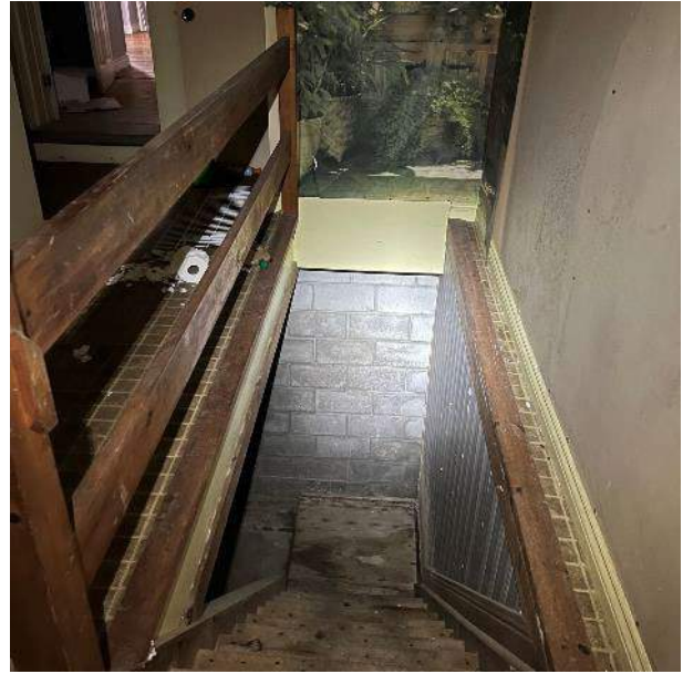
Staircase to Basement
