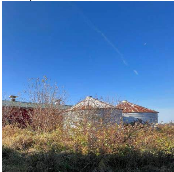
Squatter Silo Beside Drive Shed
