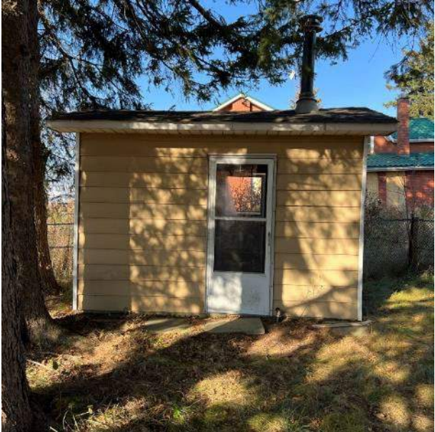
East Façade of Pool Shed
