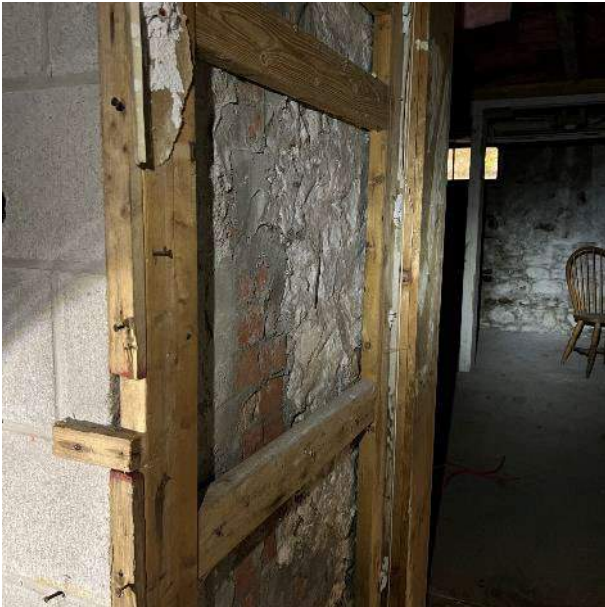
Transition between Concrete Block and Rubble Stone Foundations
