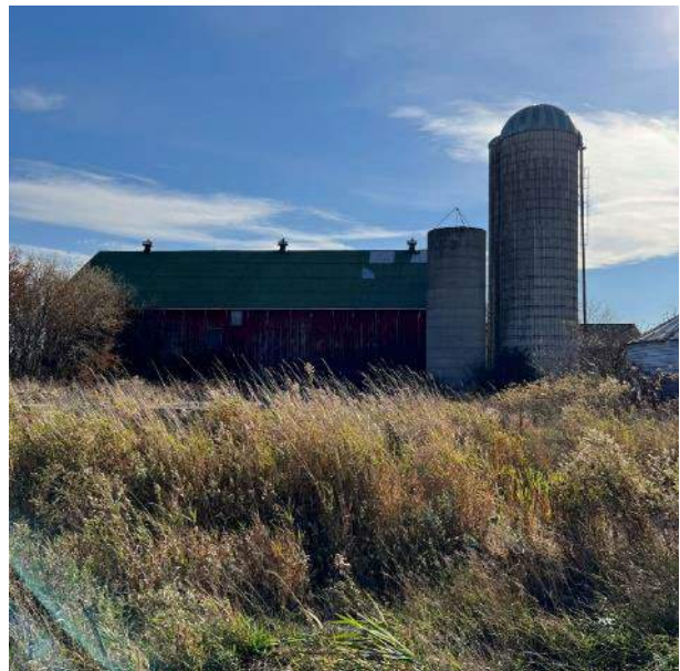
Northwest Façade of Larger Barn from a Distance
