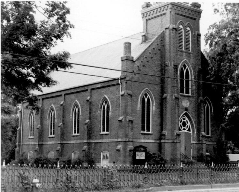
Figure 20: Norval Presbyterian Church at 499 Guelph Street, at Draper Street, c.1982 (EHS 17567)
