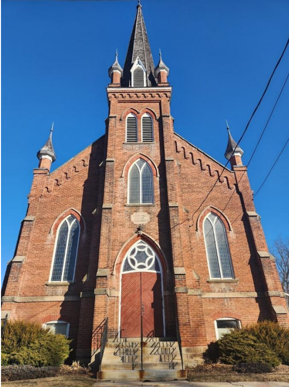
Figure 32: Front (south) elevation of Norval Presbyterian Church (Town of Halton Hills 2024)
