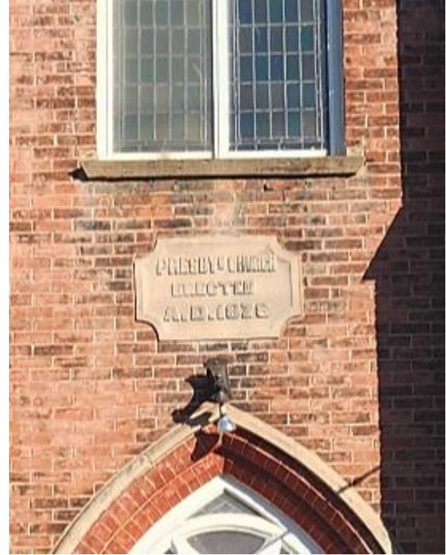
Figure 33: Detail of front (south) elevation of Norval Presbyterian Church (Town of Halton Hills 2024)
