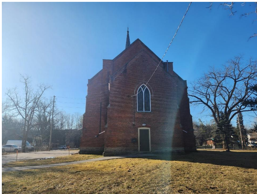
Figure 38: Rear (north) elevation of Norval Presbyterian Church (Town of Halton Hills 2024)
