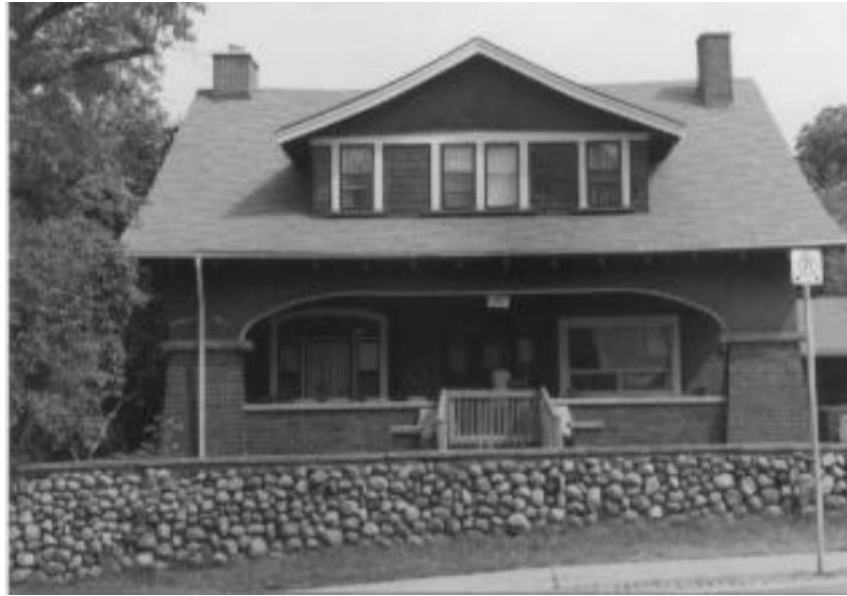
Figure 7: "The Birches" (70 Mill Street) c. 1994
