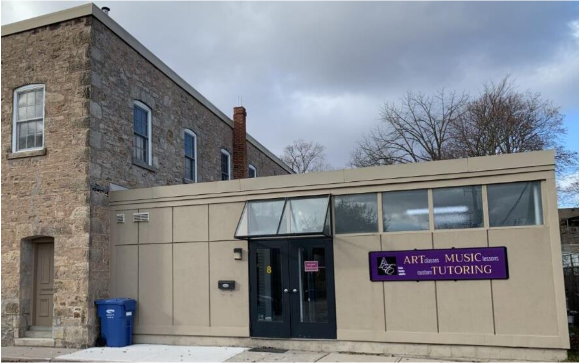
Figure 39: Partial side (northeast) elevation of the original building obscured by the one-storey concrete block addition (Town of Halton Hills 2023)
