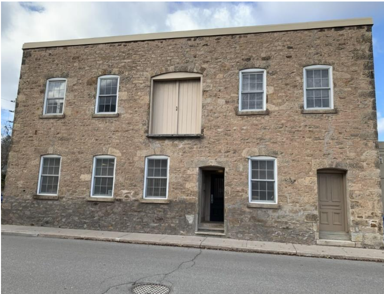
Figure 35: Primary (southeast) elevation of 8 James Street (Town of Halton Hills 2023)
