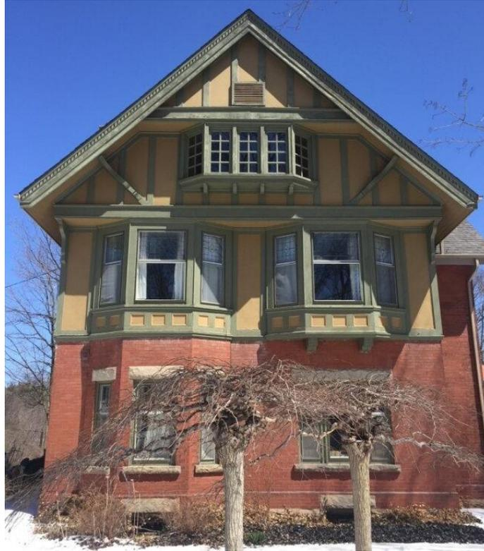
The rear (south) elevation of Barraclough House facing the Credit River is arguably the most elaborate and detailed elevation of the home, originally oriented towards the Glen Woollen Mill for its manager E.Y. Barraclough. Built into the hill, this elevation is dominated by a large covered verandah featuring elaborate wooden architectural detailing throughout.
