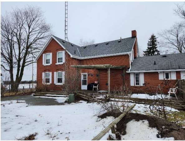
Figure 31: Looking towards the northeast elevation of the existing residence, showing the rear addition (Town of Halton Hills 2024)
