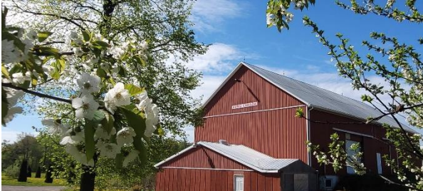
Figure 18: Spring 2022 Photographs of the subject property (AMMA Canada)
