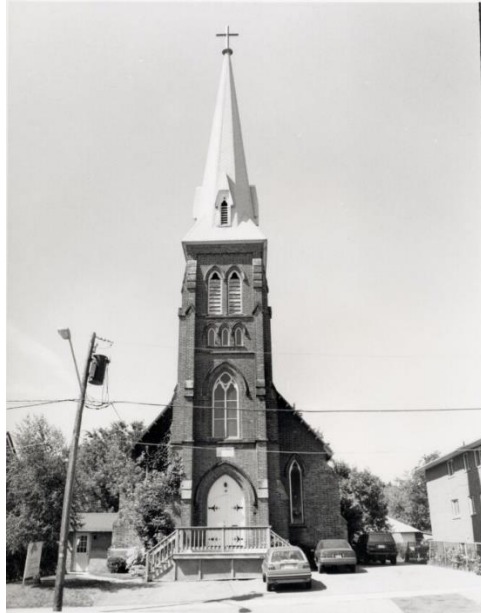
Figure 22: First Baptist Church, c.1980 (EHS 13021)
