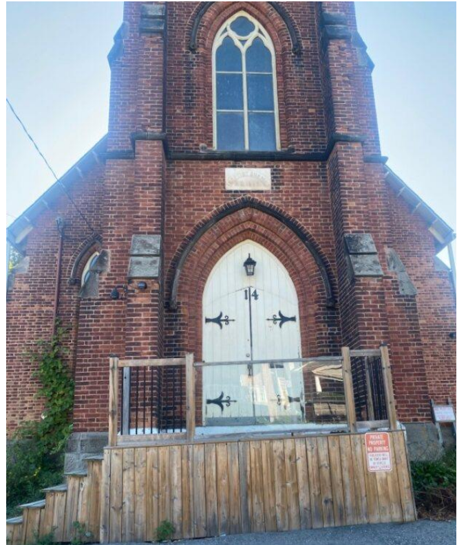
Figure 31: Detail of front (northeast) elevation of First Baptist Church at 14 Main Street South (Town of Halton Hills 2023)
