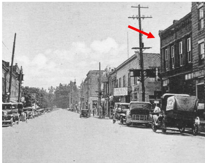
Figure 4: Main Street South c.1925. Subject property identified on the right (EHS 00094)
