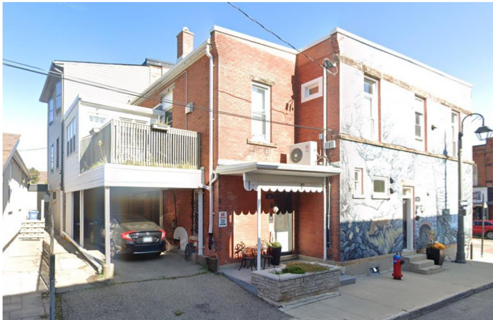
Figure 18: Rear corner of the existing building on the subject property (Google Streetview 2023)
