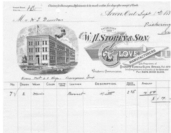
Figure 9: Sketch of W.H. Storey & Son glove factory on Bower Street on the letterhead of an invoice to Mr. H. T. Dunbar of Pickering, dated 1 Sept. 1894 (EHS00131)
