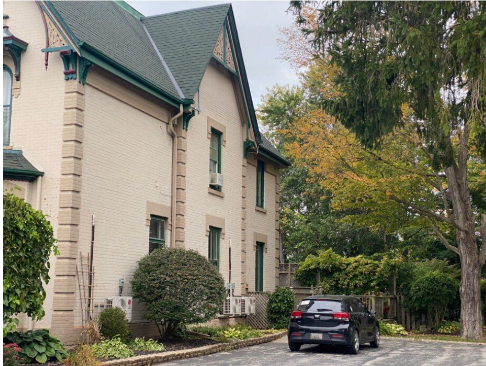
Figure 43: Side (northeast) elevation of Sunderland Villa (Town of Halton Hills 2023)
