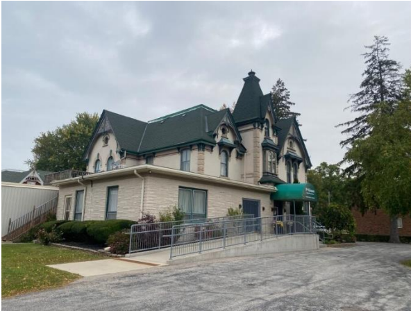
Figure 39: Southwest corner of Sunderland Villa showing the one-storey addition (Town of Halton Hills 2023)
