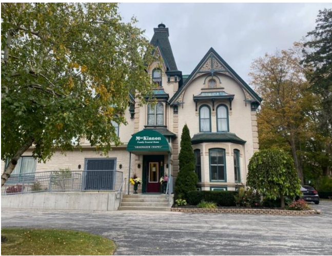
Figure 35: Partial southeast elevation of Sunderland Villa (Town of Halton Hills 2023)
