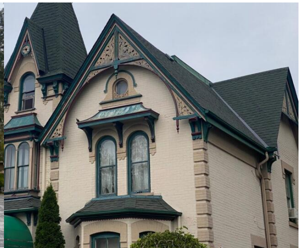
Figure 36: Detail of the southeast elevation of Sunderland Villa (Town of Halton Hills 2023)
