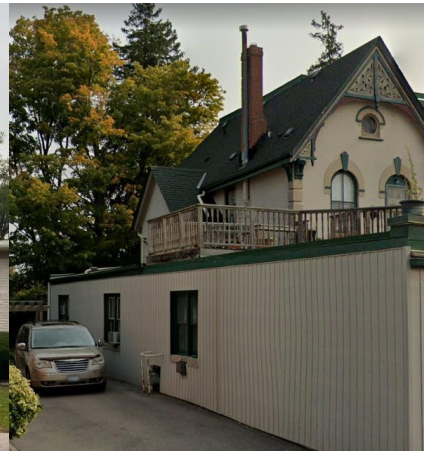
Figure 42: Rear (northwest) elevation of Sunderland Villa (Google Streetview)
