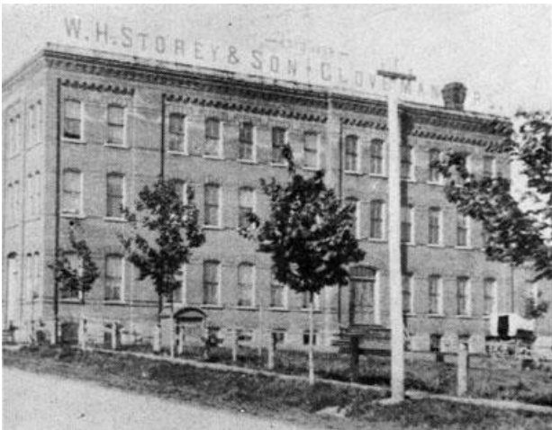
Figure 8: W.H. Storey and Son Glove Factory (EHS00383)
