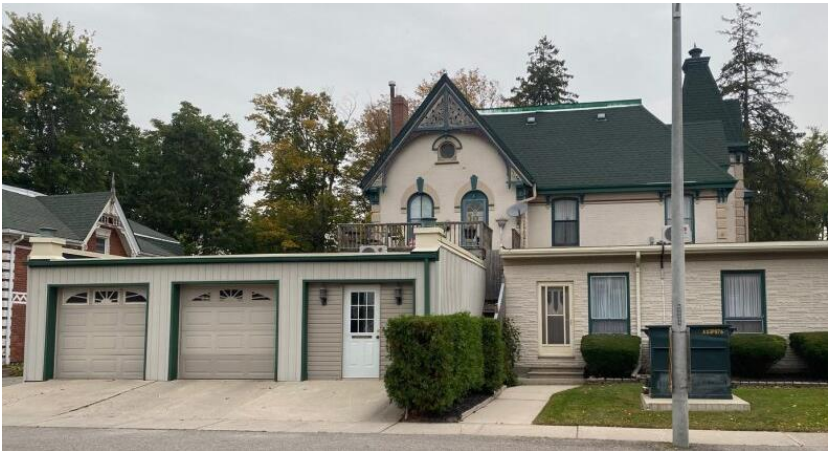
Figure 41: Southwest elevation of Sunderland Villa (Town of Halton Hills 2023)
