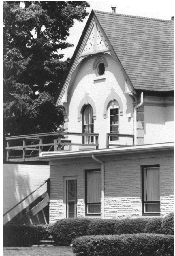
Figure 30: Detail of the west wing, c.1996 (EHS 23536)
