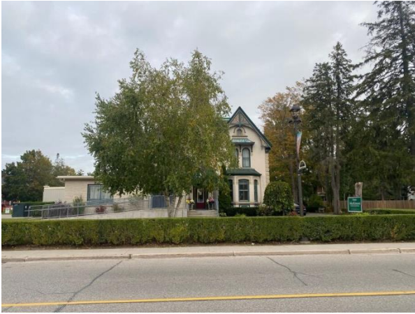
Figure 33: Looking towards the southeast elevation from Mill Street East, showing the hedge along the front property line and mature trees (Town of Halton Hills 2023)
