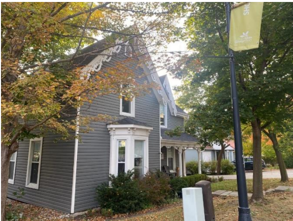
Figure 17: Detail of front elevation, 129 Main Street South (Town of Halton Hills 2023)
