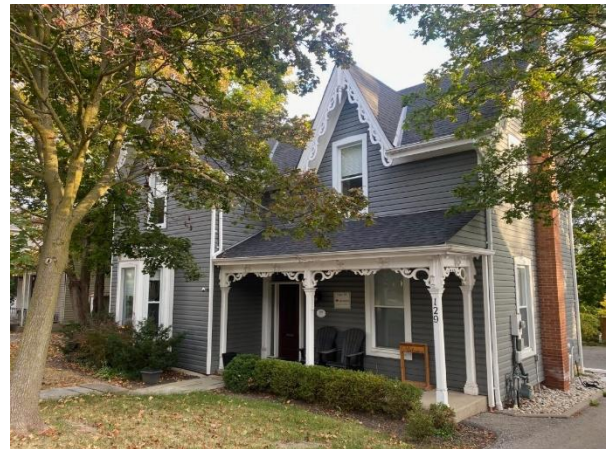
Figure 18: Detail of front elevation, 129 Main Street South (Town of Halton Hills 2023)
