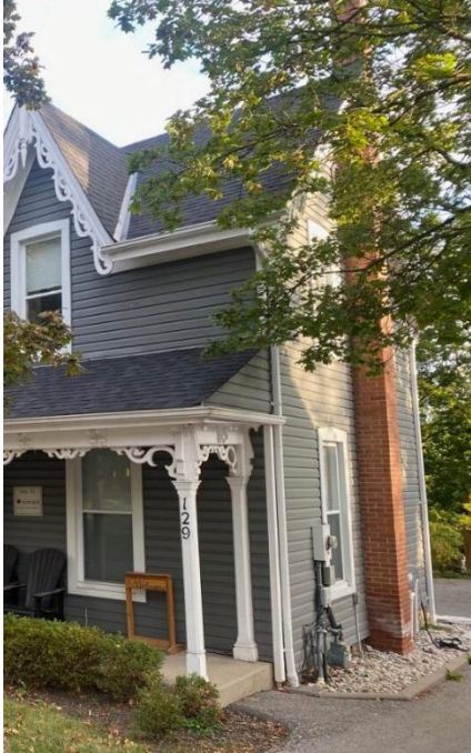
Figure 19: Partial side (south) elevation of 129 Main Street South (Town of Halton Hills 2023)
