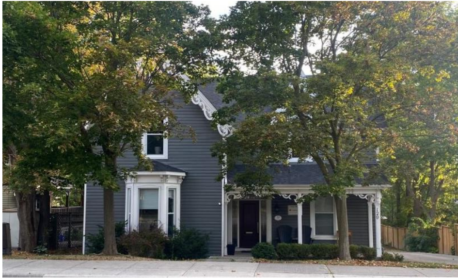
Figure 16: Front elevation of 129 Main Street South (Town of Halton Hills 2023)
