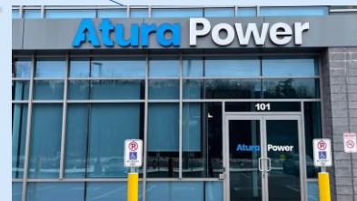
6. Oakville Head Office
