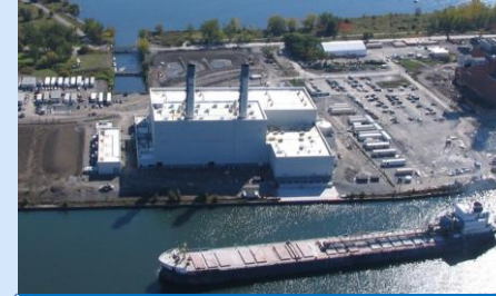
3. Portlands Energy Centre Capacity (550 MW)
