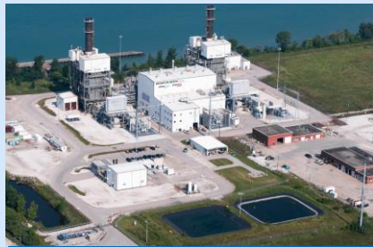
1. Brighton Beach Generating Station (570 MW)
