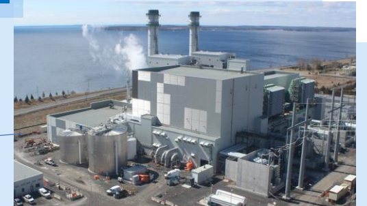
4. Napanee Generating Station (900 MW)
