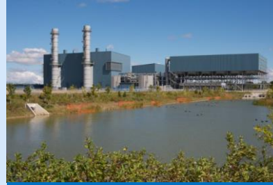
2. Halton Hills Generating Station (683 MW)
