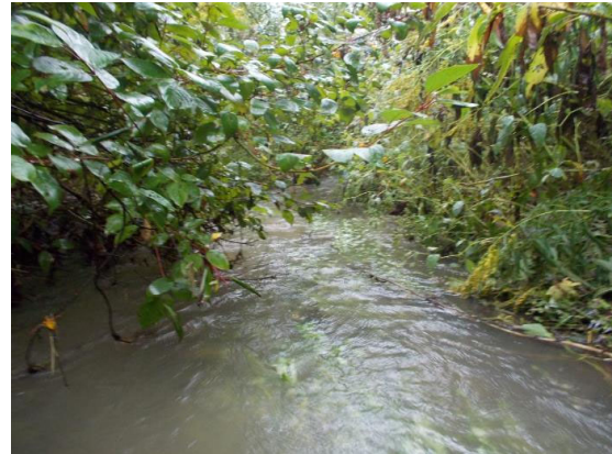
Photo 52: Station WQ4 Tyler Ave. storm outfall facing downstream, Sept. 22, 2021.
