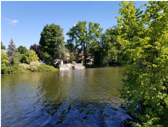
Photo 39: Polygon B - an example of hardened shoreline on north side, near the dam.
