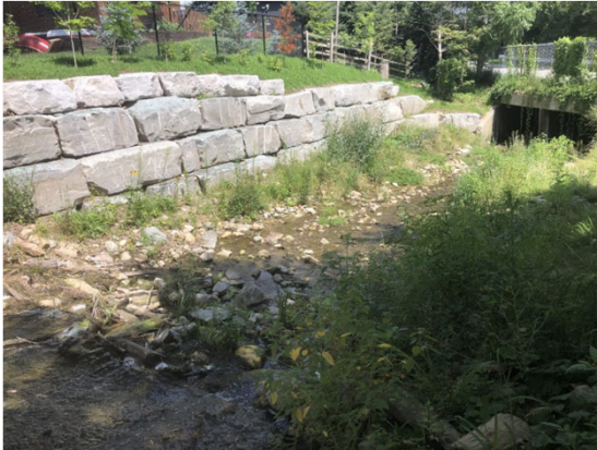
Photo 55: Station WQ6 facing downstream of dam, August 3, 2021.
