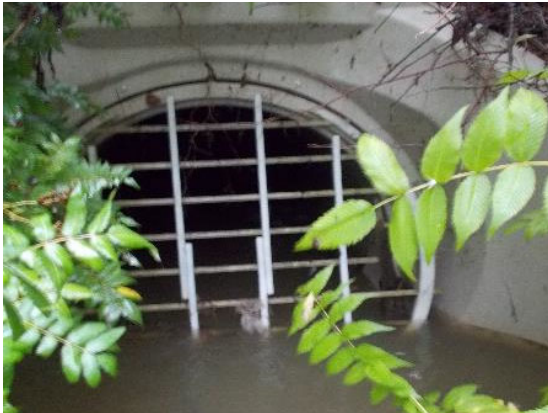
Photo 51: Station WQ4 stormwater inlet during wet weather event, Sept. 22, 2021
