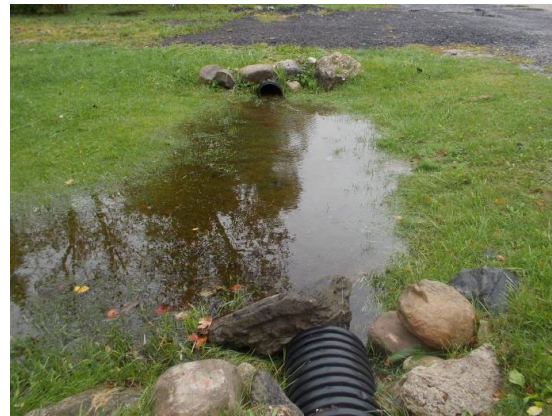
Photo 46: Station WQ2 inlet at trailer park, September 22, 2021.
