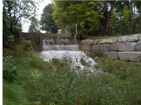
Photo 56: Station WQ6 outlet to Black Creek in wet weather, Sept. 22, 2021.
