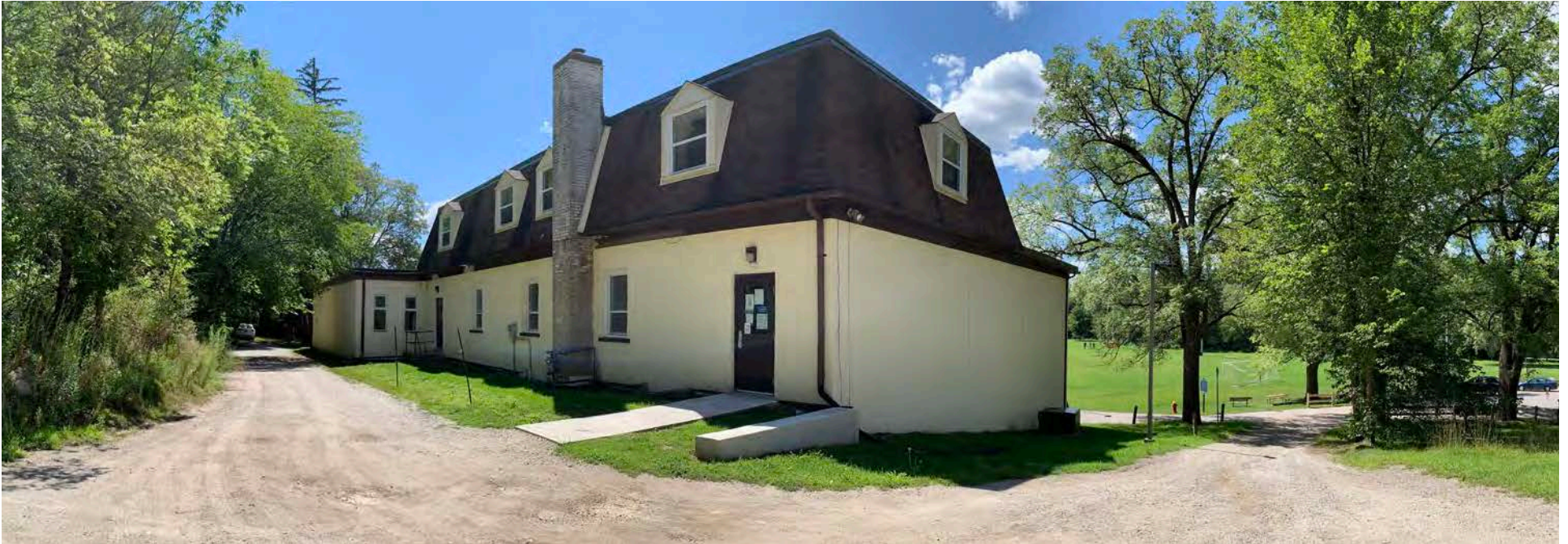
Panorama view of the rear facade of the present-day Cedarvale Community Centre Source: A composition of photos taken by ATA staff in 2021
