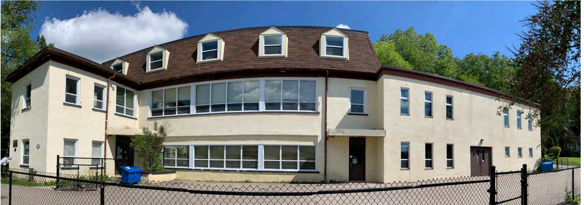
Panorama view of the front facade of the present-day Cedarvale Community Centre Source: A composition of photos taken by ATA staff in 2021
