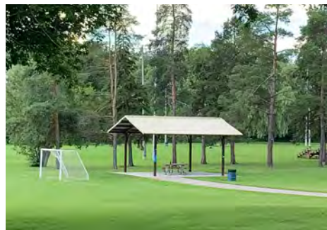
View of Existing Open Shelter in Cedarvale Park (ATA, 2021)
