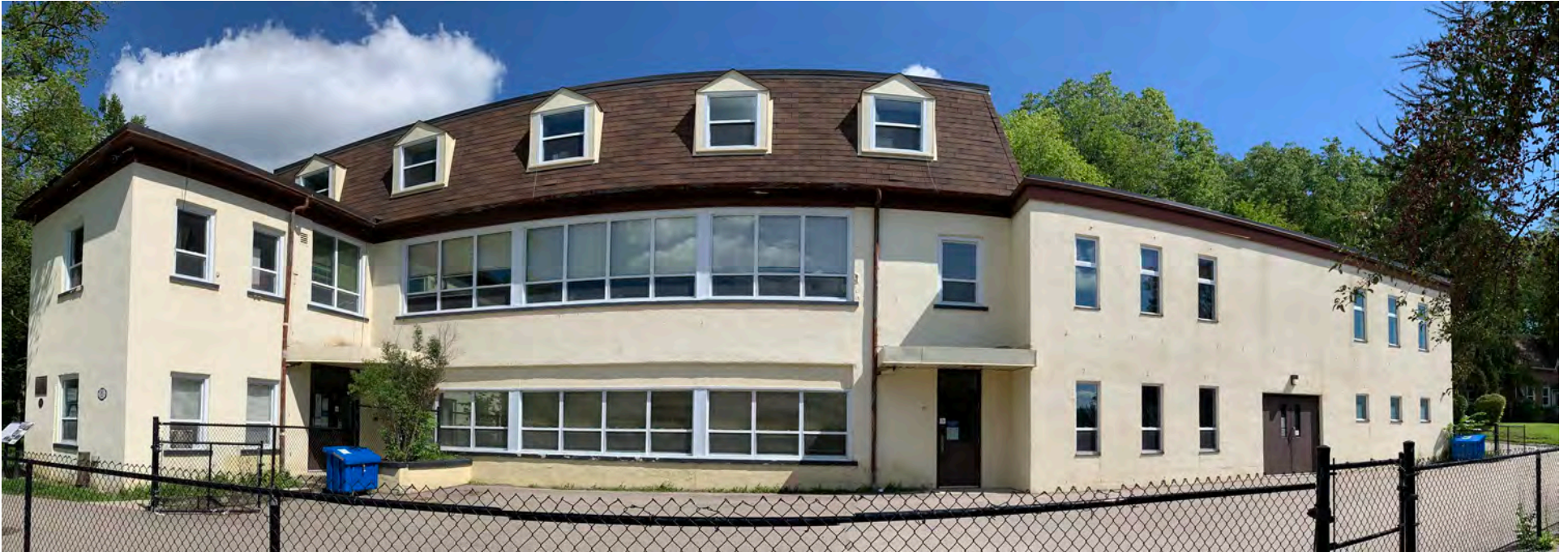
Panorama view of the present-day Cedarvale Community Centre Source: A composition of photos taken by ATA staff in 2021
