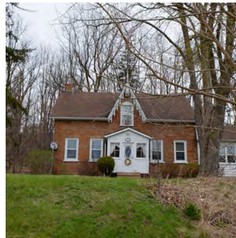
7 Use existing historical resource building such as Freeman-Bradley House and Cedarvale Cottage.
