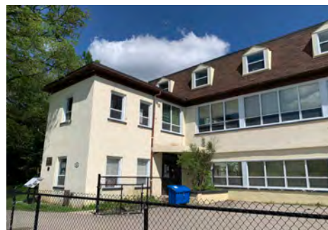
Front View of Existing Community Centre (ATA, 2017)
