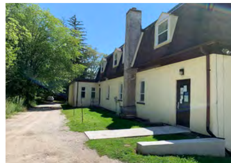
Rear View of Existing Community Centre (ATA, 2021)
