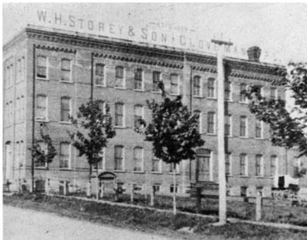
Figure 3: W.H. Storey and Son Glove Factory (EHS00383)
