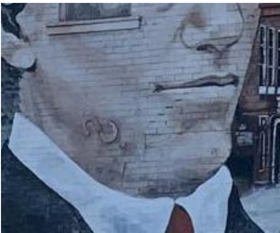
Figure 24: S-shaped wall anchor along the east elevation (Town of Halton Hills 2023)
