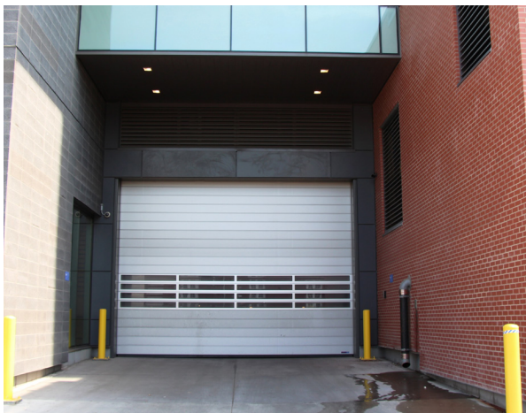
A service and loading area within the building structure.
