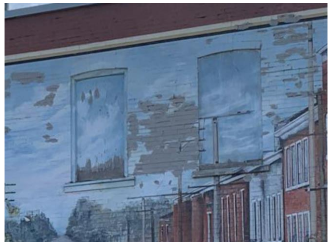
Figure 25: In-filled window openings at the upper storey, 26 Guelph Street (Town of Halton Hills 2023)
