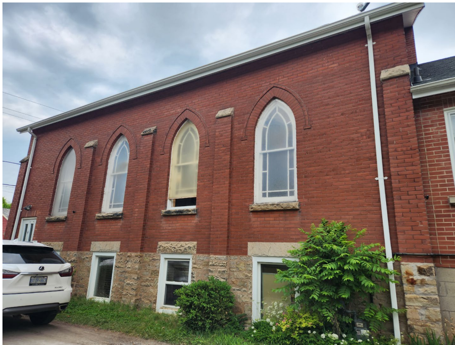
Figure 19: South elevation (Town of Halton Hills 2023)
