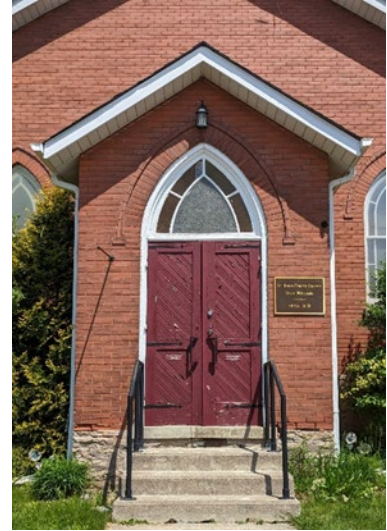
Figure 16: Front door and vestibule (J.M. Rowe June 2023)
