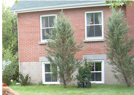
Figure 20: 2006 view of north side of the 1962 addition. J.M. Rowe photo
