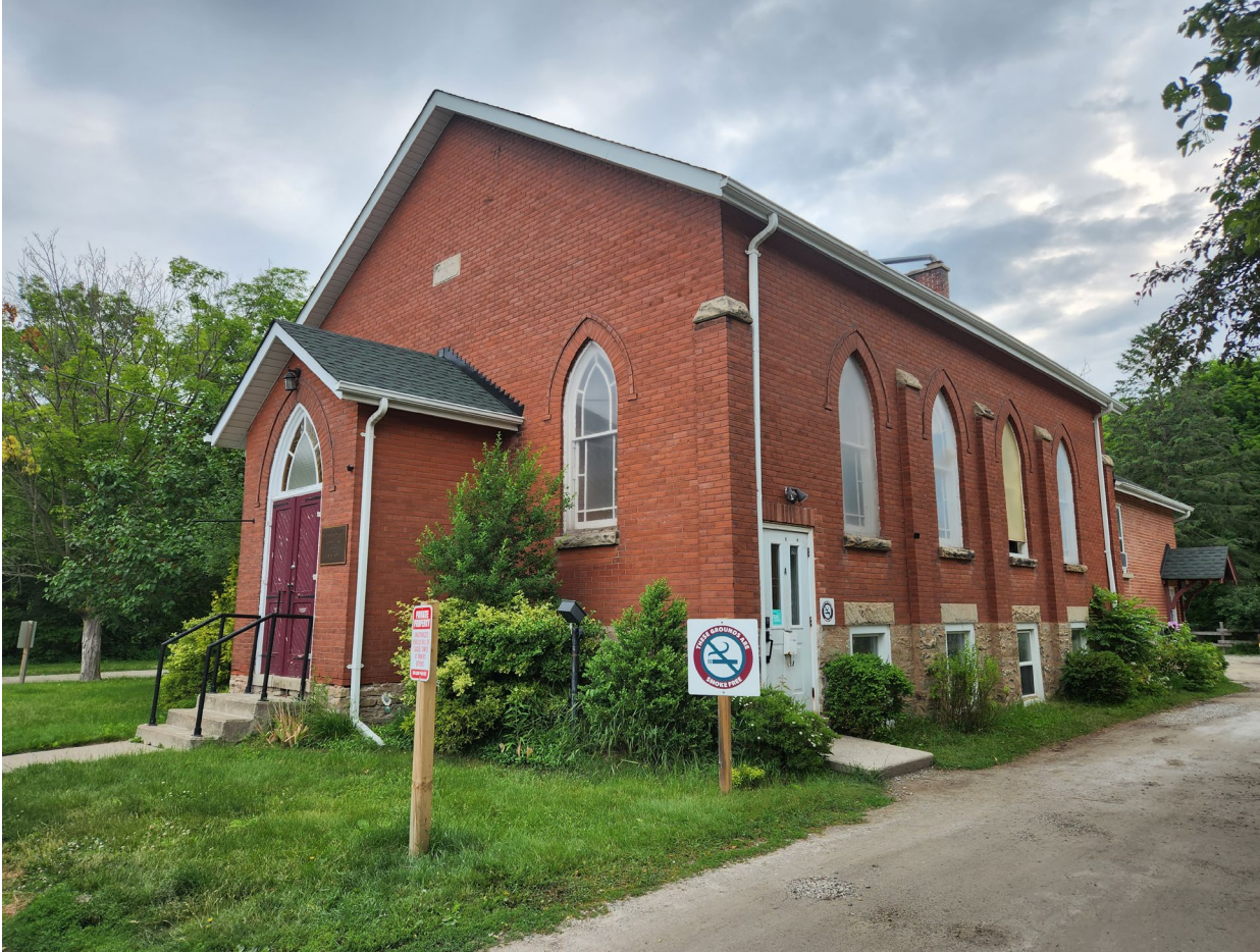
Figure 17: Looking northeast towards the existing building (Town of Halton Hills 2023)
