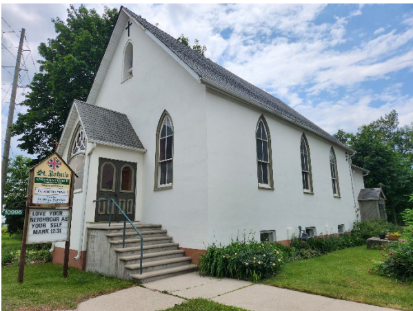
Figure 30: Northwest corner of St. John's Anglican Church (Town of Halton Hills 2023)
