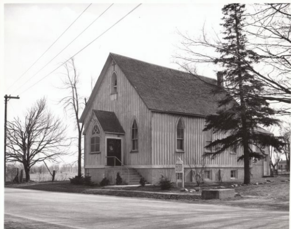
Figure 12: St. John's Anglican after basement construction (Courtesy of The Georgetown Vault)
