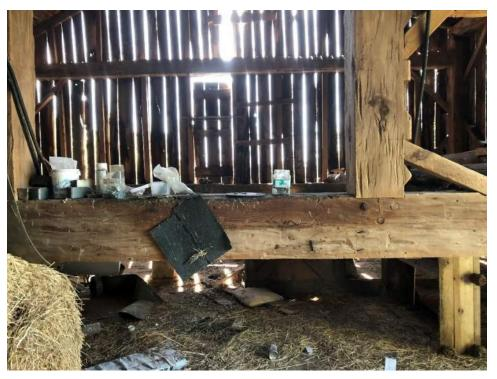
Image 86: View of the mortise and tenon joinery and hand-hewn beams.
