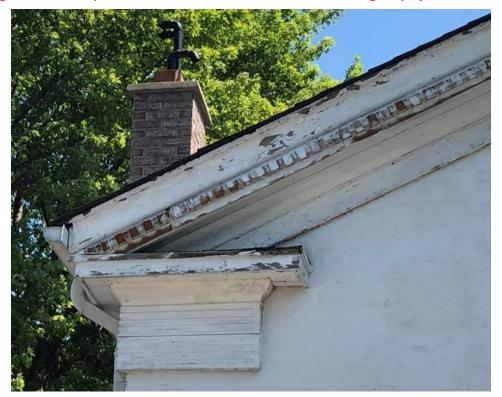
Image 101: Detail view of the dentil detailing, revealing the polyurethane material where the exterior coating has worn away.
