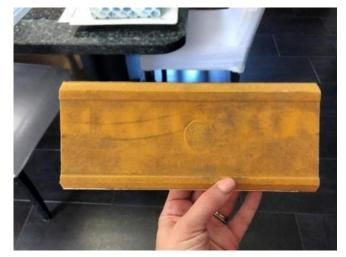
Image 100: View of the back of the dentil detailing revealing the polyurethane material.
