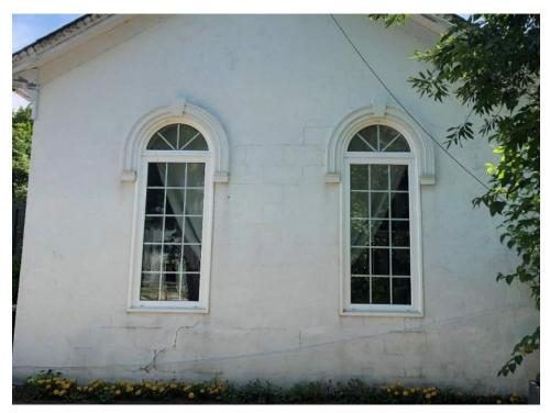
Image 27: View of the windows on the west elevation of the west addition, note the faint lines in the stucco displaying the concrete block construction.
