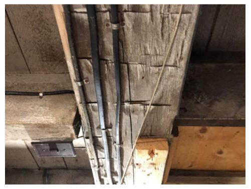
Image 64: Detail of a hand-hewn beam in the basement.
