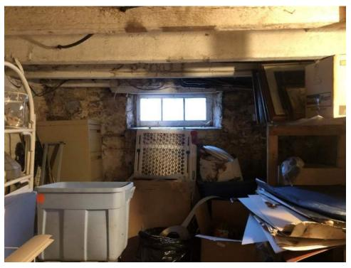
Image 63: View of the stone foundation walls and a wood window.
