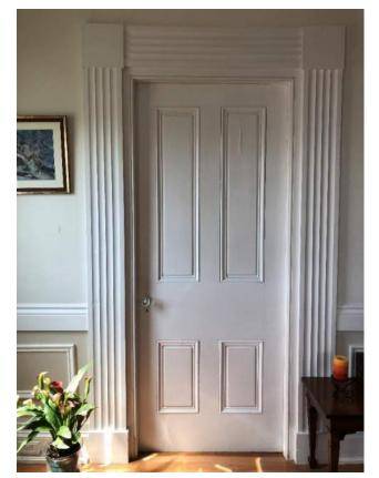
Image 41: View of the paneled door and fluted door surround leading to the small room on the west end of the original part of the house's first storey.
