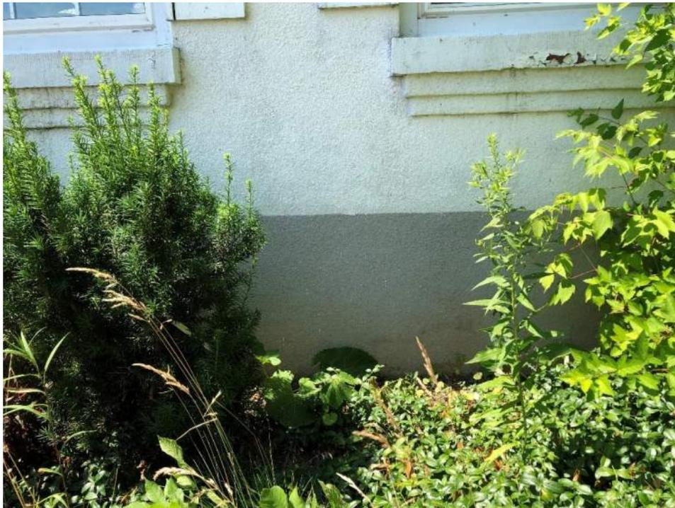
**Image 12: Detail of the stuccoed foundation that is painted grey (this is consistent with the foundation treatment on all elevations).**
