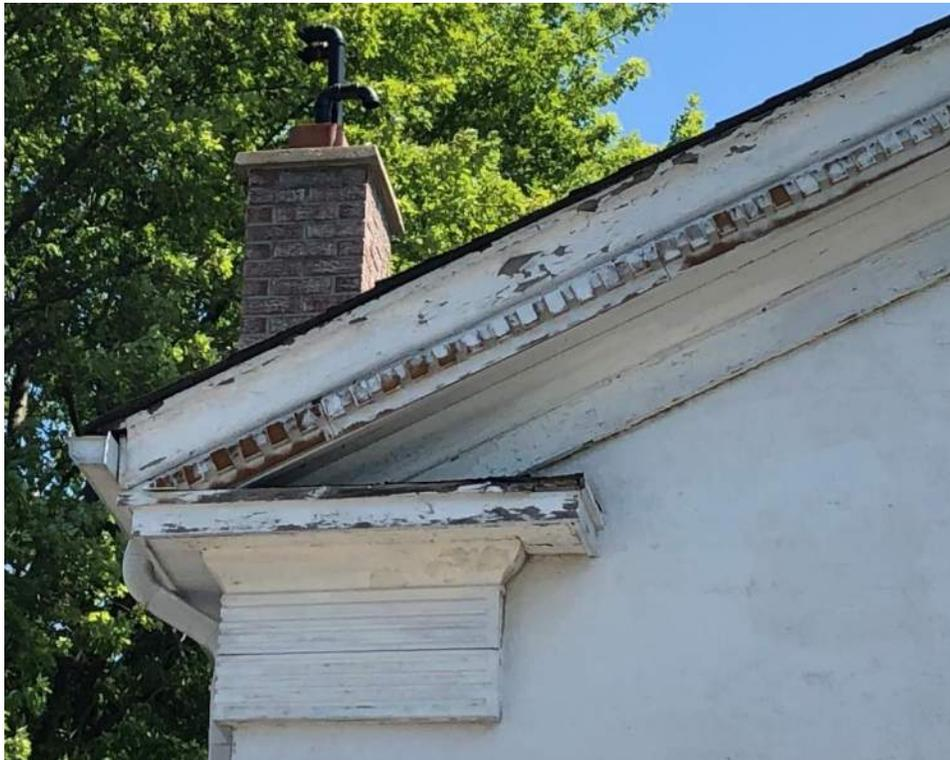
**Image 101: Detail view of the dentil detailing, revealing the polyurethane material where the exterior coating has worn away.**
