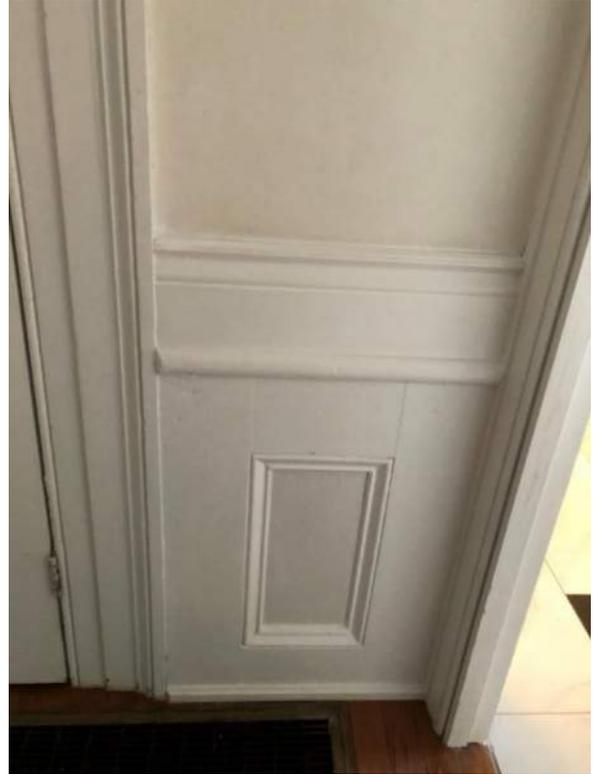
**Image 34: View of the recessed wall paneling.**
