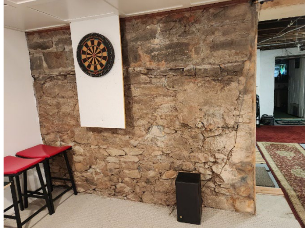
Figure 28: Rubble stone foundation within interior basement, 68 Bower Street (Town of Halton Hills 2023)
