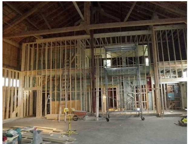
Figure 25: The installation of new walls and stairs for new amenities and second floor access c. 2010-2015 (Globe Productions)
