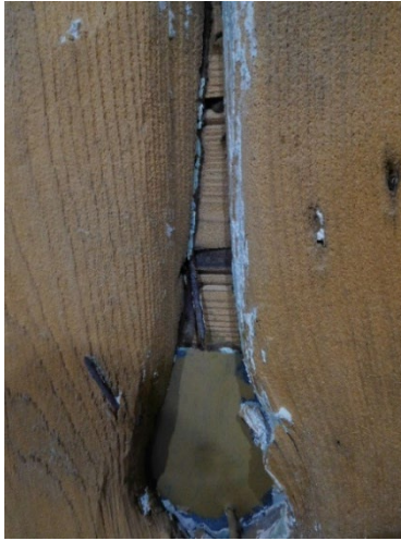
Figure 51: Parts of the original tongue-in-groove siding beneath the barn-boards and foamboard insulation (Town of Halton Hills 2022)
