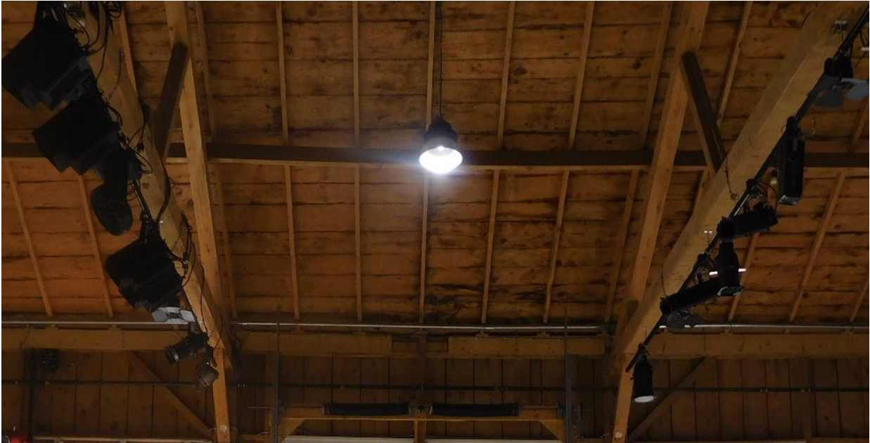
Figure 55: The barnboard roof. Modern installations such as lighting fixtures and stage lights have been installed into the timber frame (Town of Halton Hills 2022)
