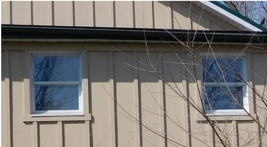
Figure 47: Double Hung Windows are located along the northeast elevation of the Armoury building (Town of Halton Hills 2022)
