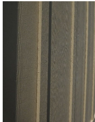
Figure 52: Fibre-cement (James Hardie) exterior siding, done in a board-batten style (Town of Halton Hills 2022)
