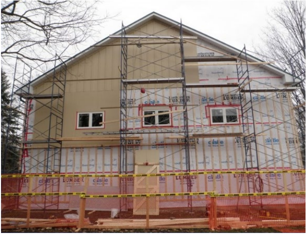
Figure 22: Installation of the James Hardie fibre cement cladding, reminiscent of the original board-batten cladding (Globe Productions 2010)
