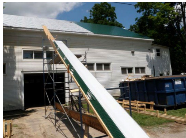
Figure 21: Old roof being replaced with green steel c. 2010 (Globe Productions)
