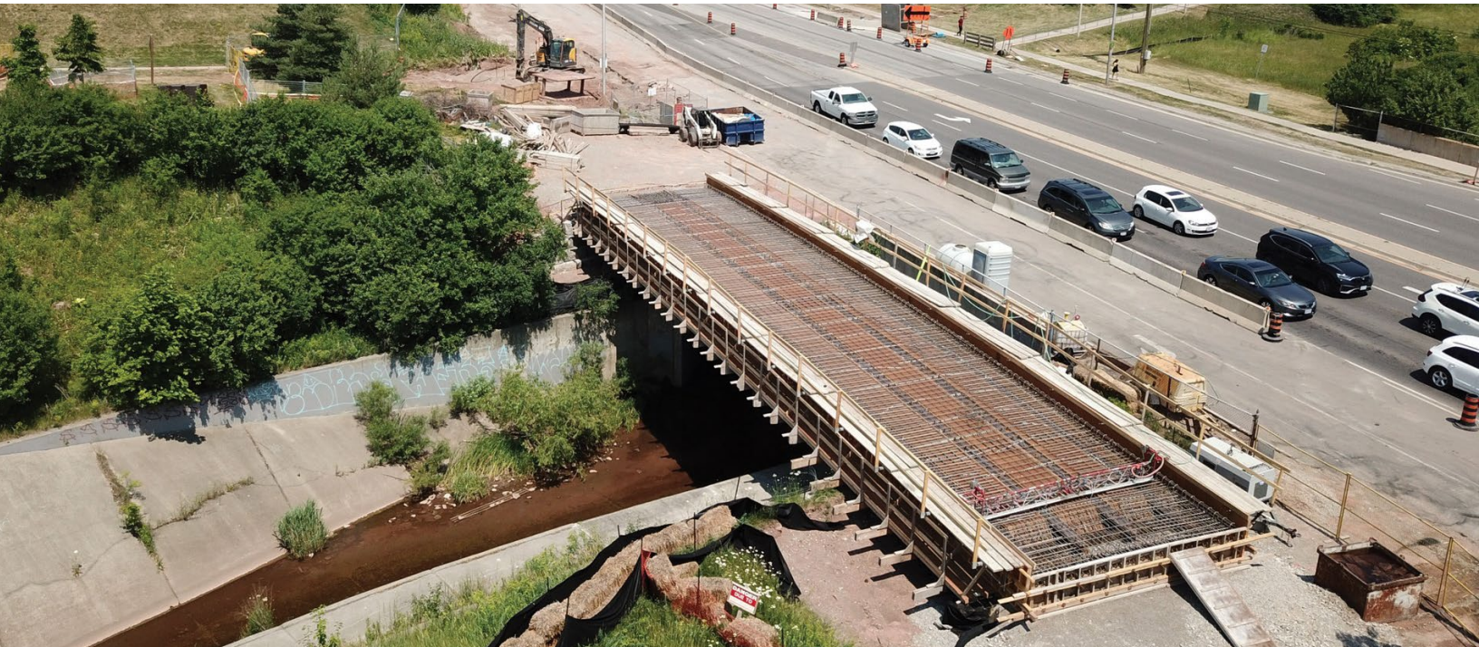
Trafalgar road project
