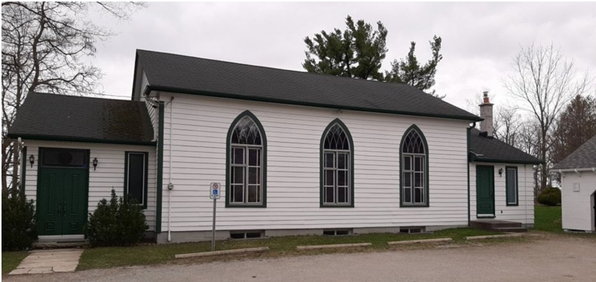
Figure 7: North side showing the three sections. L to R: front vestibule (entrance), sanctuary (original), back vestry with washrooms (Denny 2022)
