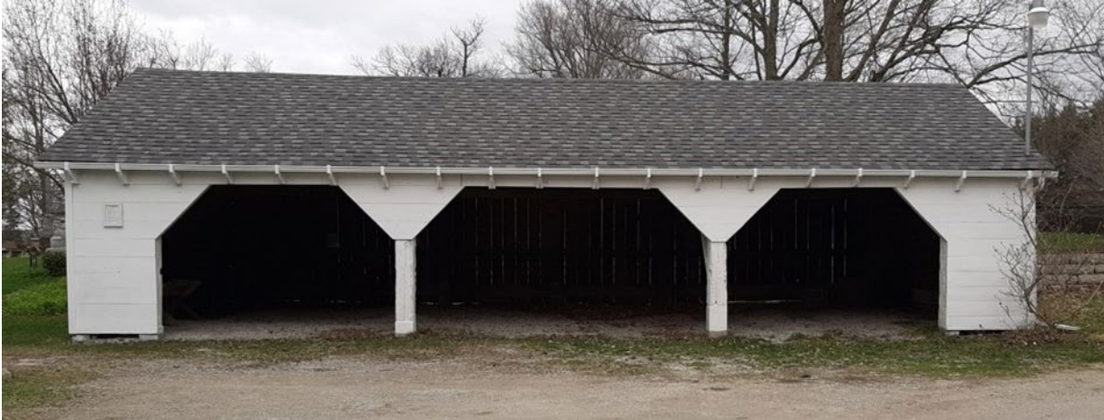
Figure 14: Front view of the shed facing northeast. (Denny 2022)
