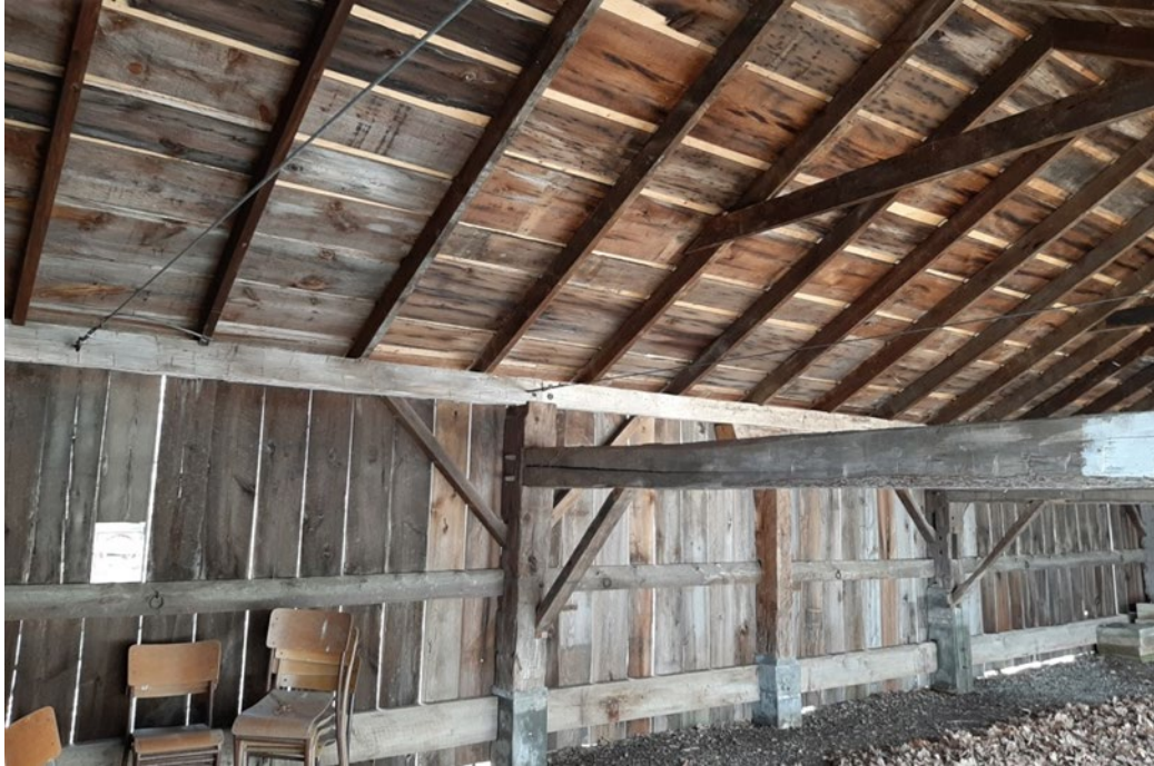
Figure 15: Traditional post and beam construction (Denny 2022)
