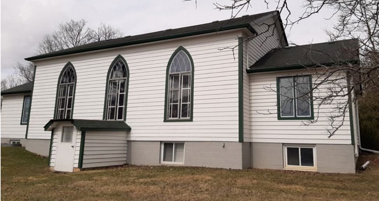
Figure 8: South side showing the main structure, additions, and exterior exit from the basement (Denny 2022)
