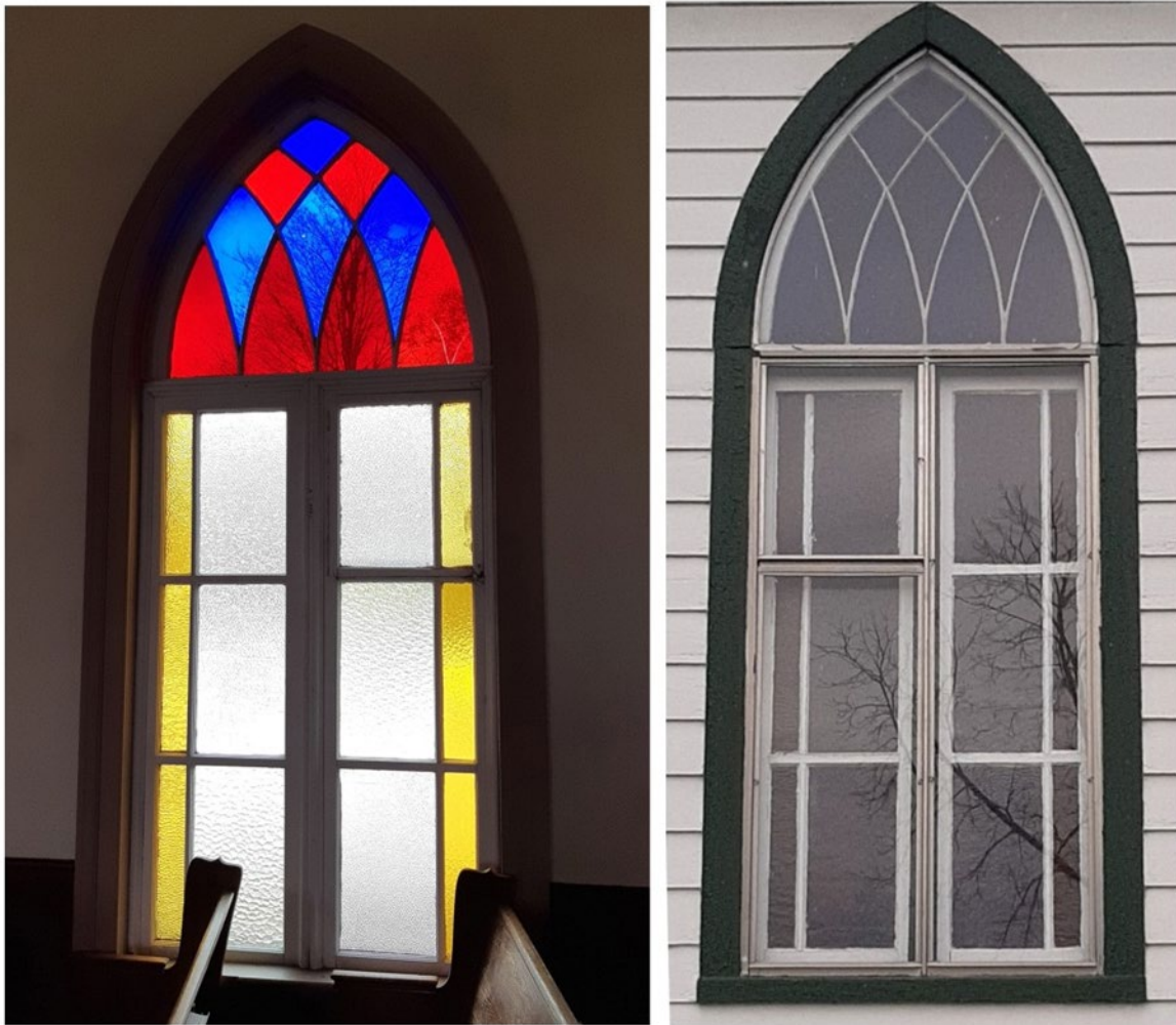
Figure 10: Inside view displays the rich colours and mullions, while aluminum storms protect the outside of the windows (Denny 2022)
