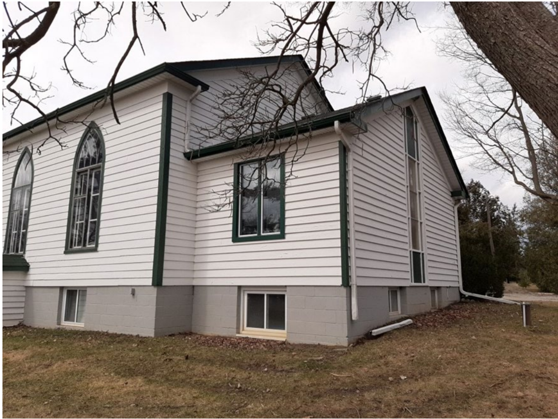
Figure 9: South-east side displaying basement and exterior features including eave returns, corner trim, gables, barge board and window placement (Denny 2022)
