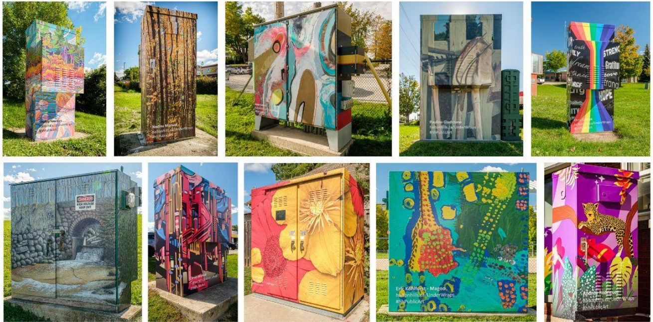
Figure 2: Completed Under Wraps Cabinets
