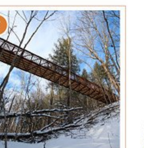
Regan Ridge Bridge
