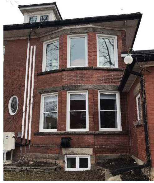
Figure 18: 76 Bower Street, side elevation detail showing projecting bay with flat-headed window openings at the first and second storey with stone sills and lintels (Town of Halton Hills 2022)
