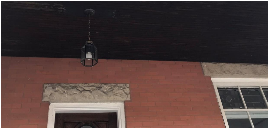
Figure 13: 76 Bower Street, front porch detail showing wood-panelled ceiling, stone lintels above the entrance and window, and stained glass transom (Town of Halton Hills 2022)
