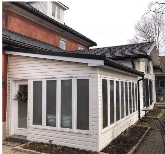
Figure 20: 76 Bower Street, rear one-storey frame addition with vinyl siding (Town of Halton Hills 2022)
