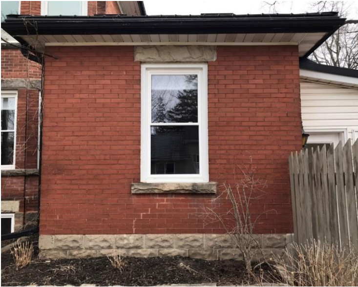
Figure 17: 76 Bower Street, side elevation detail showing flat-headed window opening with stone lintel and sill, red brick exterior and block stone foundation (Town of Halton Hills 2022)
