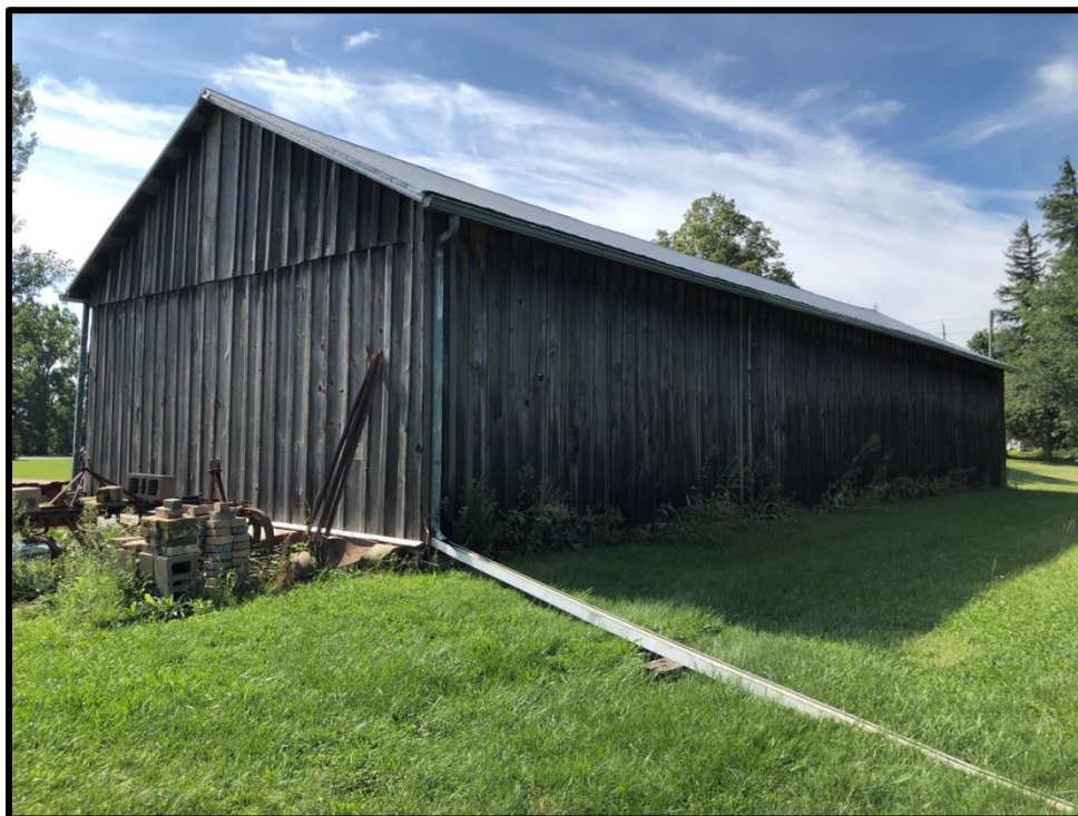
Image 26: Board and Batten Exterior Cladding on the North Elevation (Photo taken August 30, 2021; Facing South)
