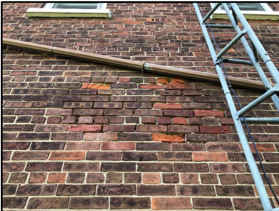
Image 16: Brick Bond Deterioration on Northwest Elevation (Photo taken August 30, 2021; Facing South)
