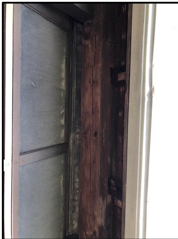
Image 22: Hand Hewn Timbers Visible at Outbuilding Entrance (Photo taken August 30, 2021; Facing North)
