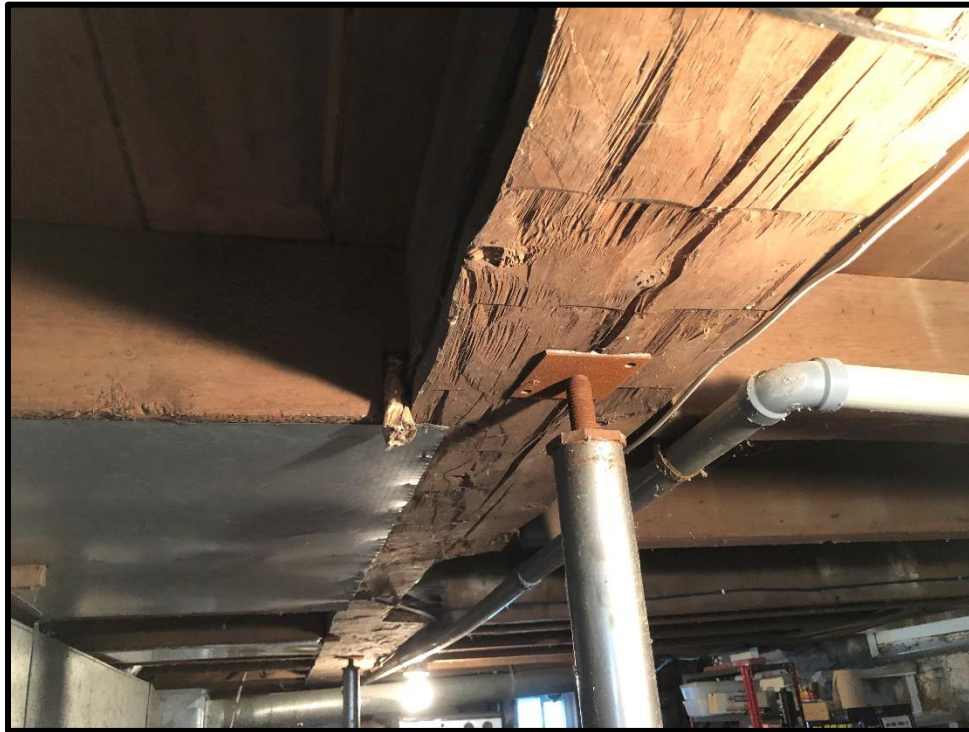
Image 61: Hand Hewn Beams Visible in Basement (Photo taken August 30, 2021)
