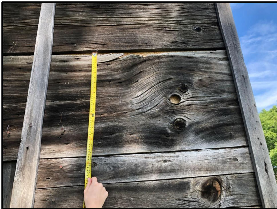
Image 30: Shed Structure – Constructed of Wide Wooden Boards (Photo taken August 30, 2021; Facing Northwest)
