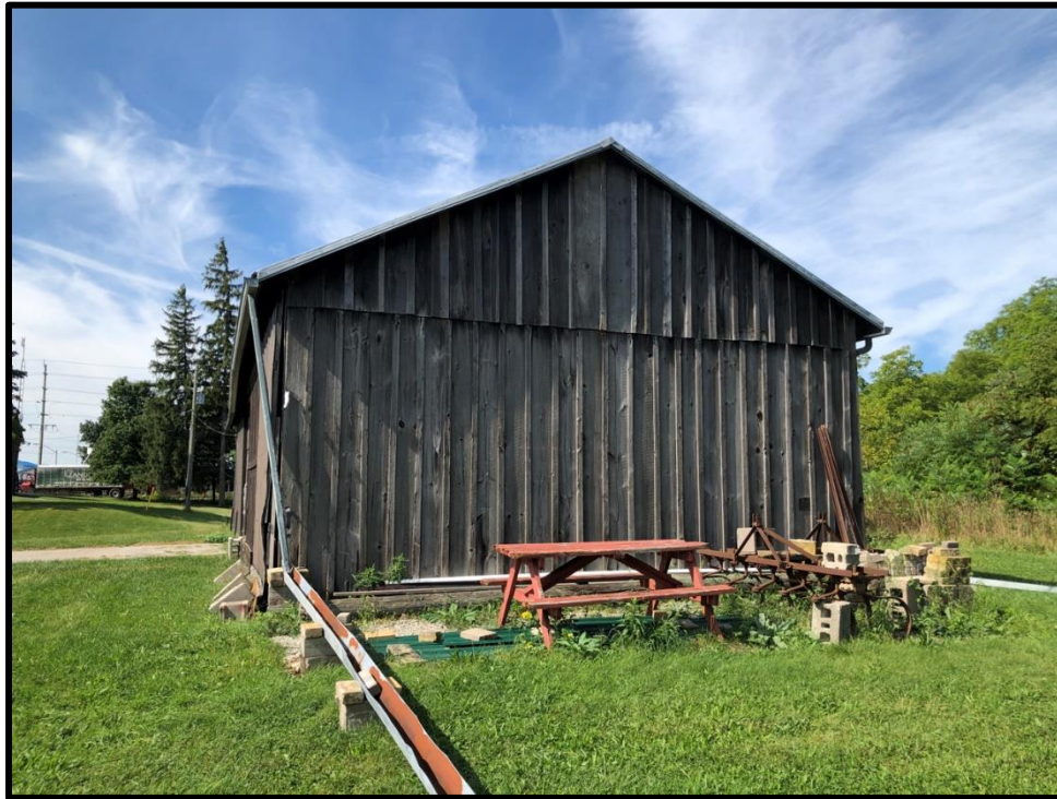
Image 25: Board and Batten Exterior Cladding on East Elevation (Photo taken August 30, 2021; Facing Southwest)
