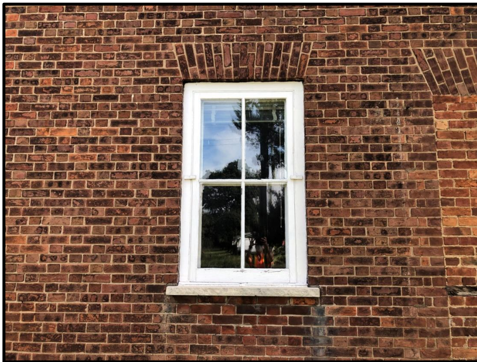
Image 6: Flat or Jack Brick Arches on Window Openings (Photo taken August 30, 2021; Facing East)
