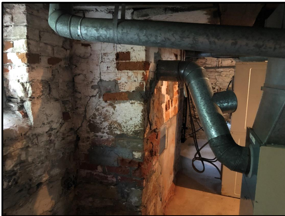
Image 64: Brick Chimney Showing Signs of Brick Deterioration (Photo taken August 30, 2021)
