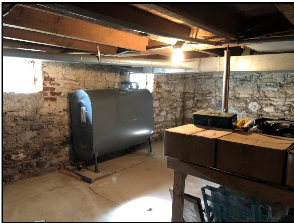
Image 62: Basement with Concrete Floor and Fieldstone Foundation with Brick Infill at Windows (Photo taken August 30, 2021)
