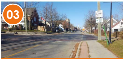
03 Location on a minor arterial road
