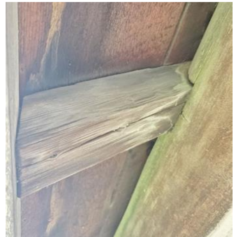
Figure 18: The top log notched to support the rafter (J.M. Rowe 2021)
