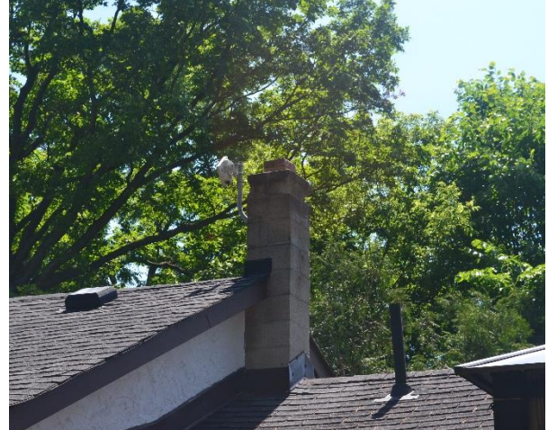
Figure 13: Original cement block chimney in the center of the gable at the south end of the building (Town of Halton Hills 2021)
