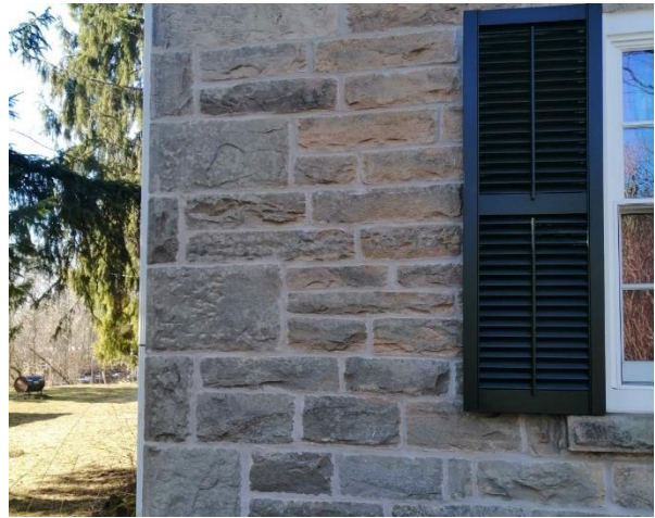
Figure 27: Ford House, detail of quoining at front elevation (Town of Halton Hills 2021)
