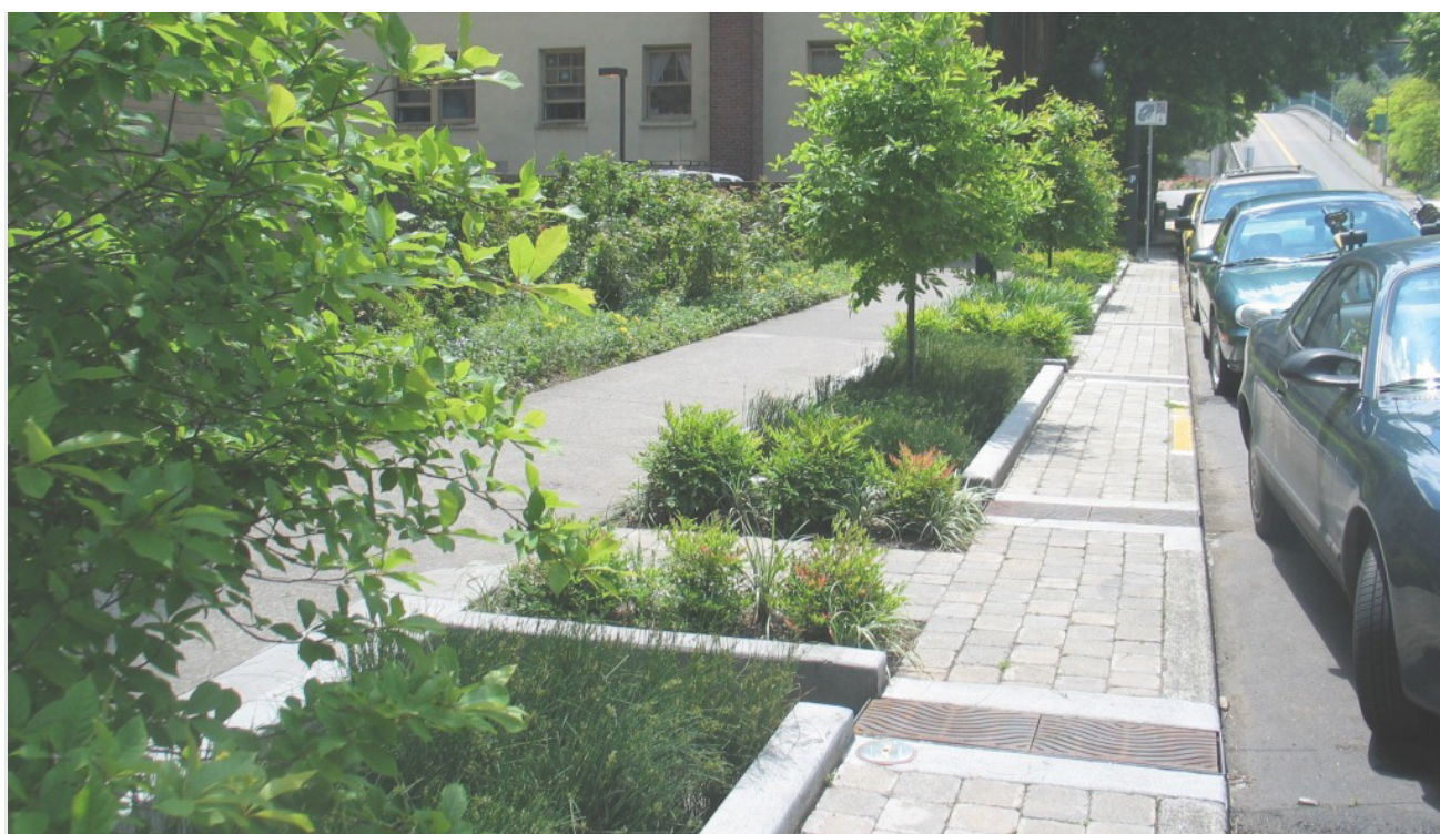
Figure 54: Planted bioswale to mitigate stormwater runoff
