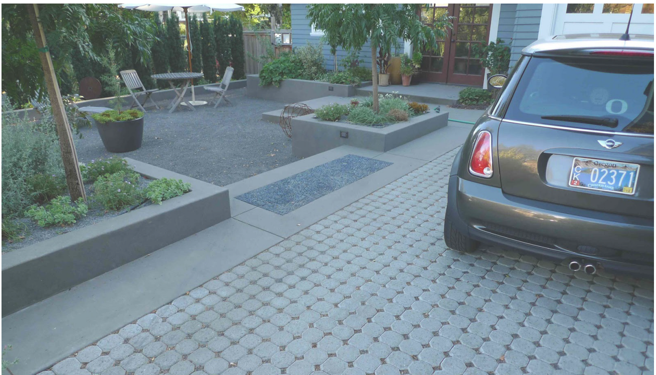
Figure 52: Permeable surface materials use on driveway are preferable
